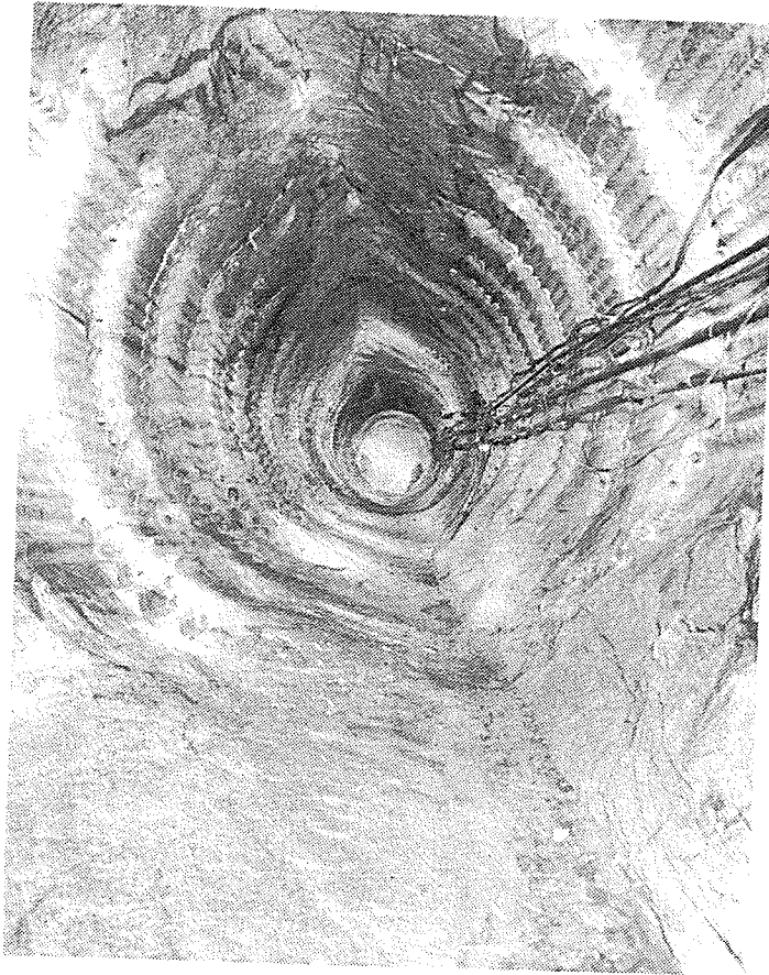
Figure 5.16: Mine-by test tunnel after excavation. The notch geometry observed in the roof and floor was caused by the spalling process.
