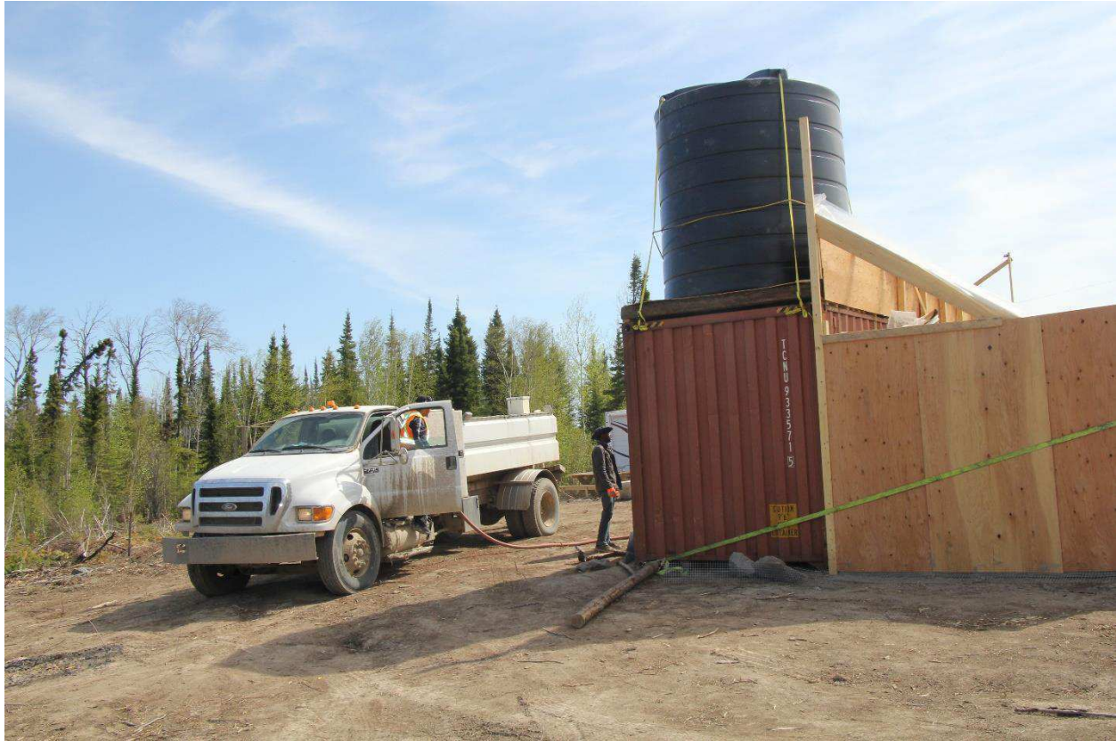
Figure 4. 8: Cistern system being filled by water truck
