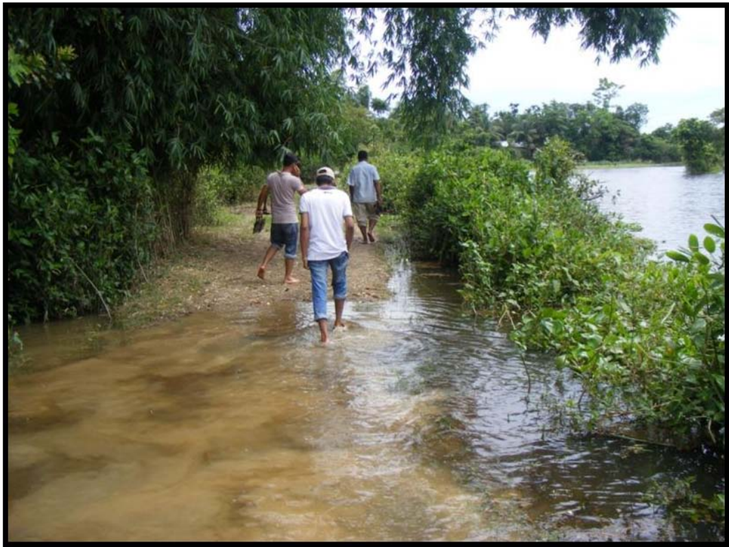
Plates 3.1: Rising water inundating the rural road during May 2011.
