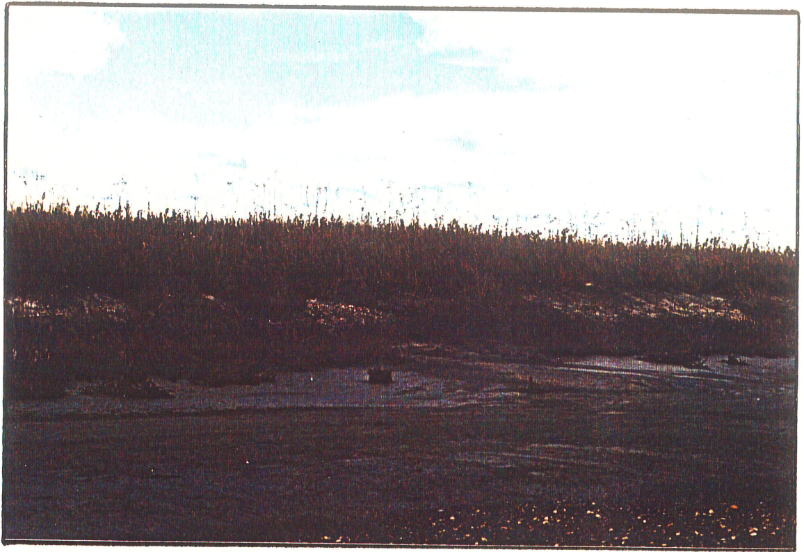
Plate No. 17: Slumping along field border into the ditch.
