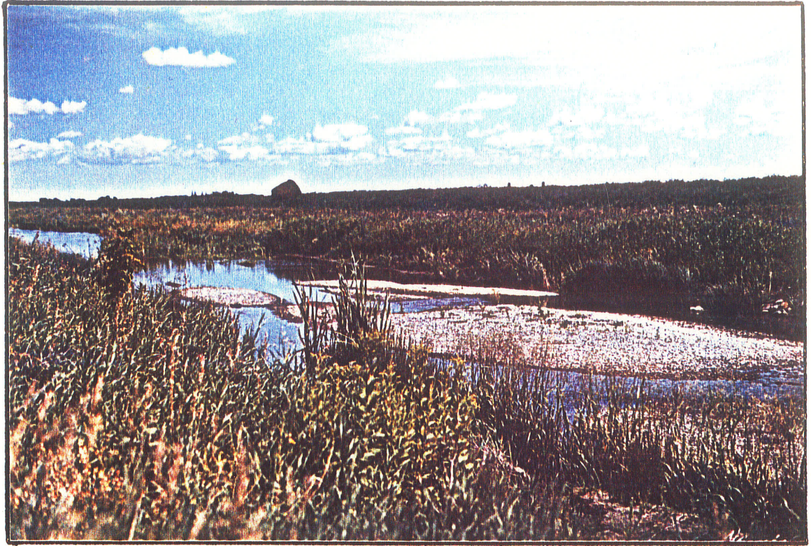
Plate No. 2: Reeve Drain prior to shale removal.
