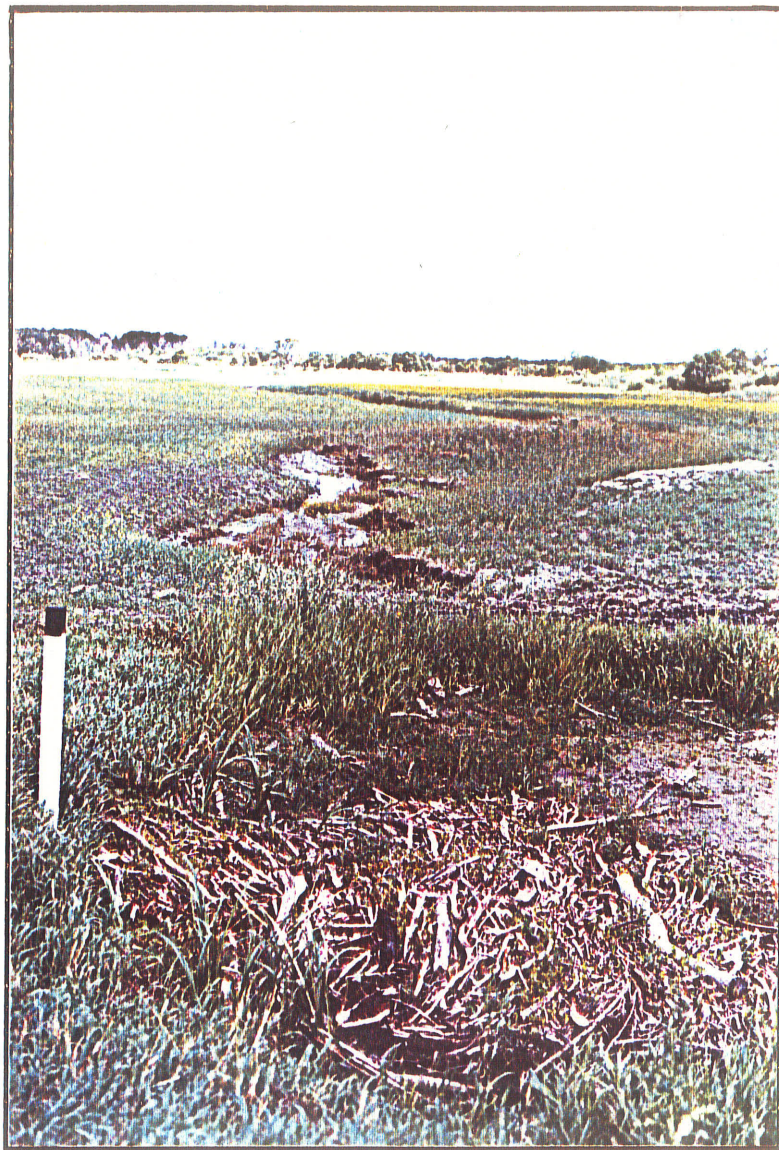
Plate No. 1: Gullying of field due to overtopping of a drainage ditch. Shale deposits reduced ditch capacity causing overtopping.
