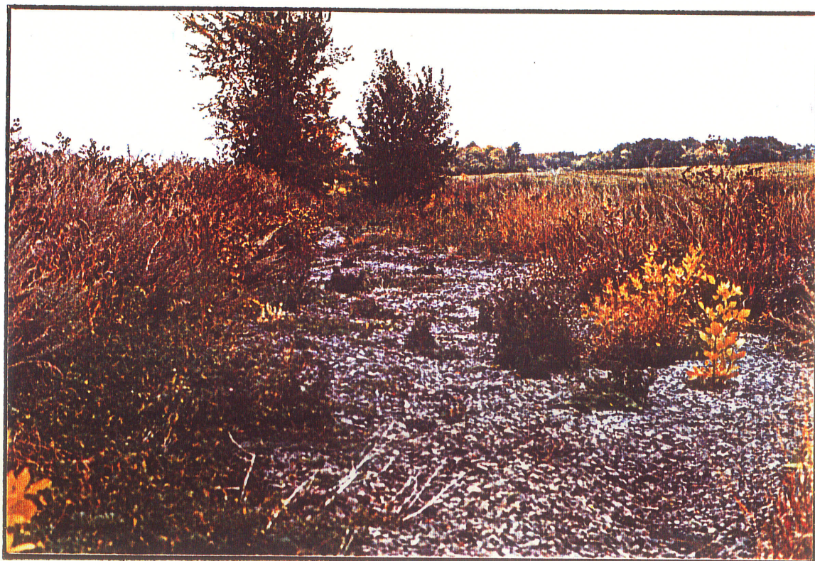
Plate No. 8: Shale deposits reduced capacity of Bearistow Drain, pictured here, and overtopping caused deposits shown in previous plate.
