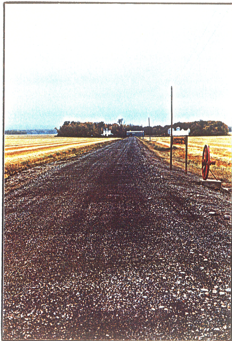
Plate No. 6: Shale driveway on a farm near the Reeve Drain.
