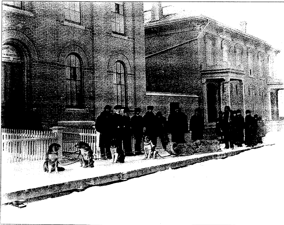
Fig. 38 Wooden sidewalk as local improvement, Winnipeg (PAM N9724) (Hamilton, 14)
