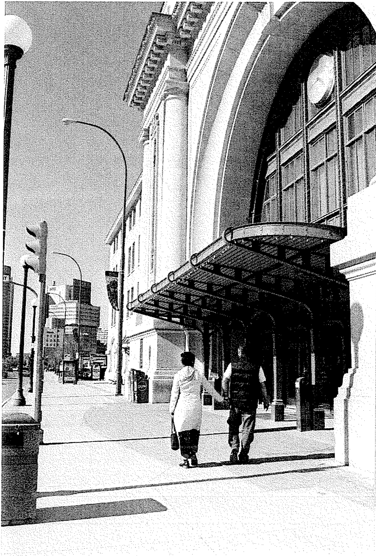
Fig. 92 Canopy encroachment Via Rail Station, Main Street, Winnipeg (author).
