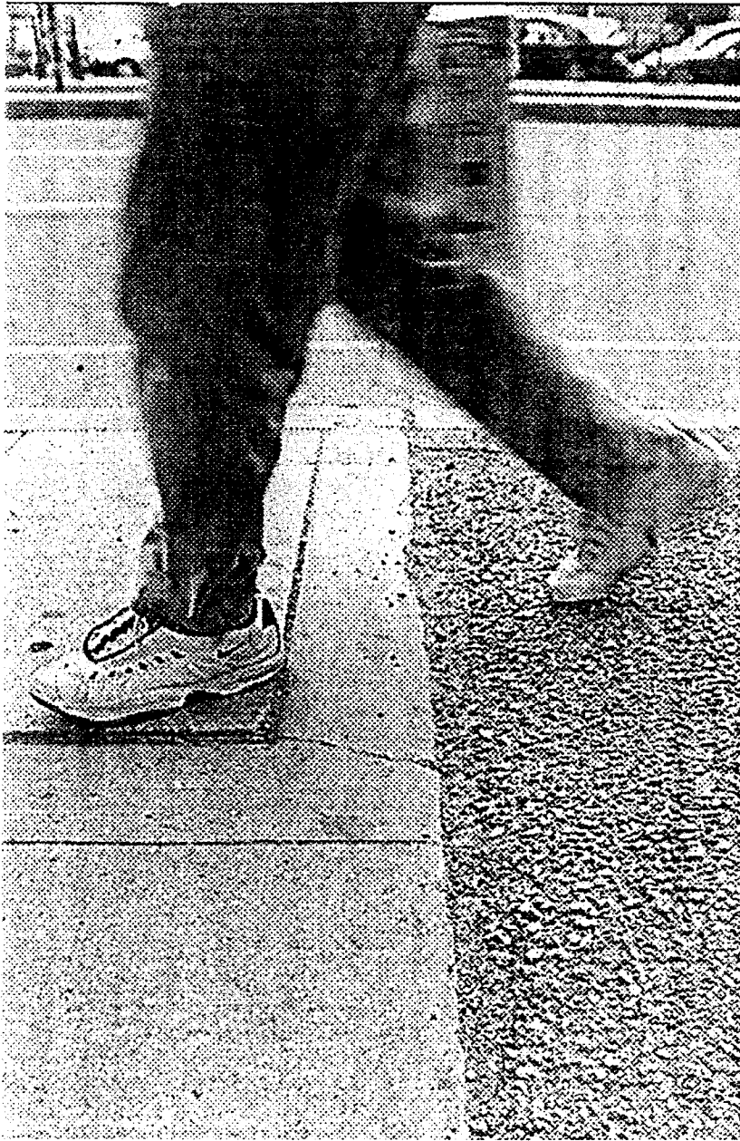
Fig. 14 Cracks in the Sidewalk System photo by Donald Weber for The Globe and Mail, Toronto.
