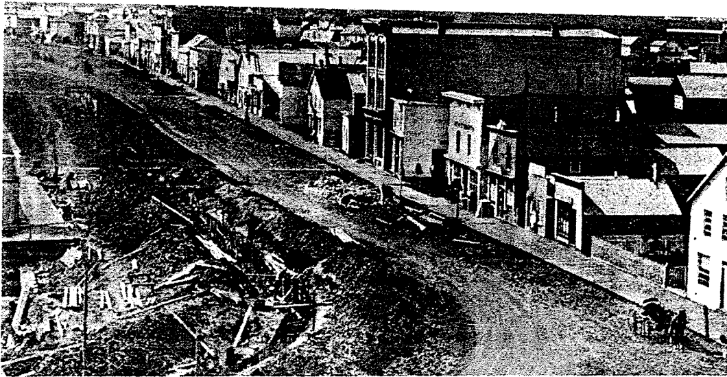
Fig. 35 Main Street sewer construction, 1875 (Winnipeg 100, 4)
