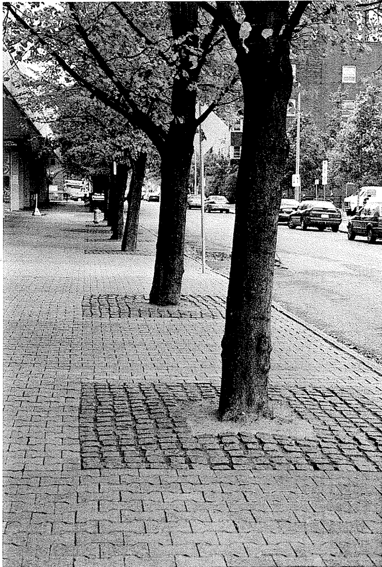
Fig. 137 Permeability of the sidewalk landscape and healthy street trees, Elgin Street, Ottawa (author).
