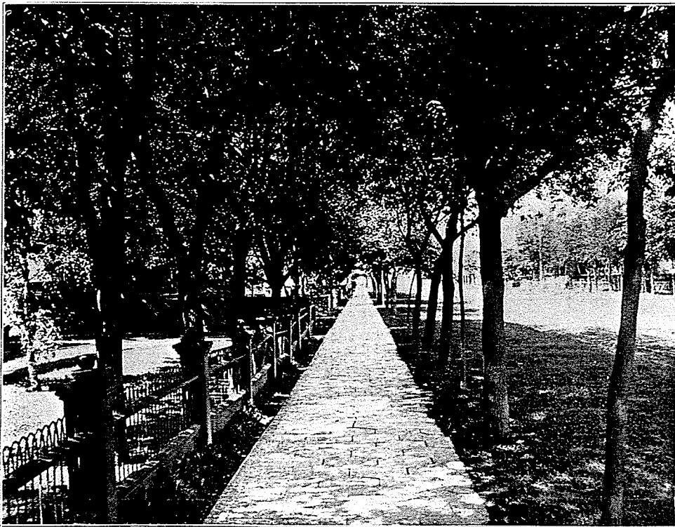
Fig. 37 Cement tile sidewalk Donald Street looking north, 1895 (Winnipeg Images)
