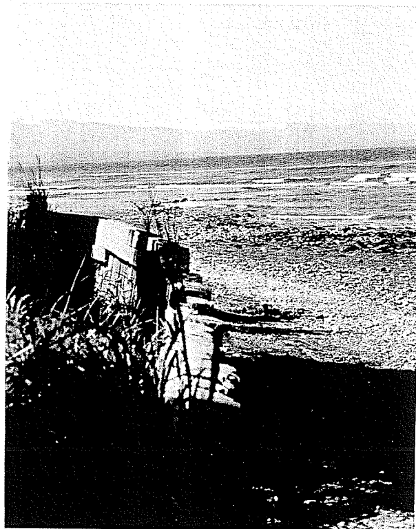
Photo 34: Breakwater on Beach, M. Mitchell
