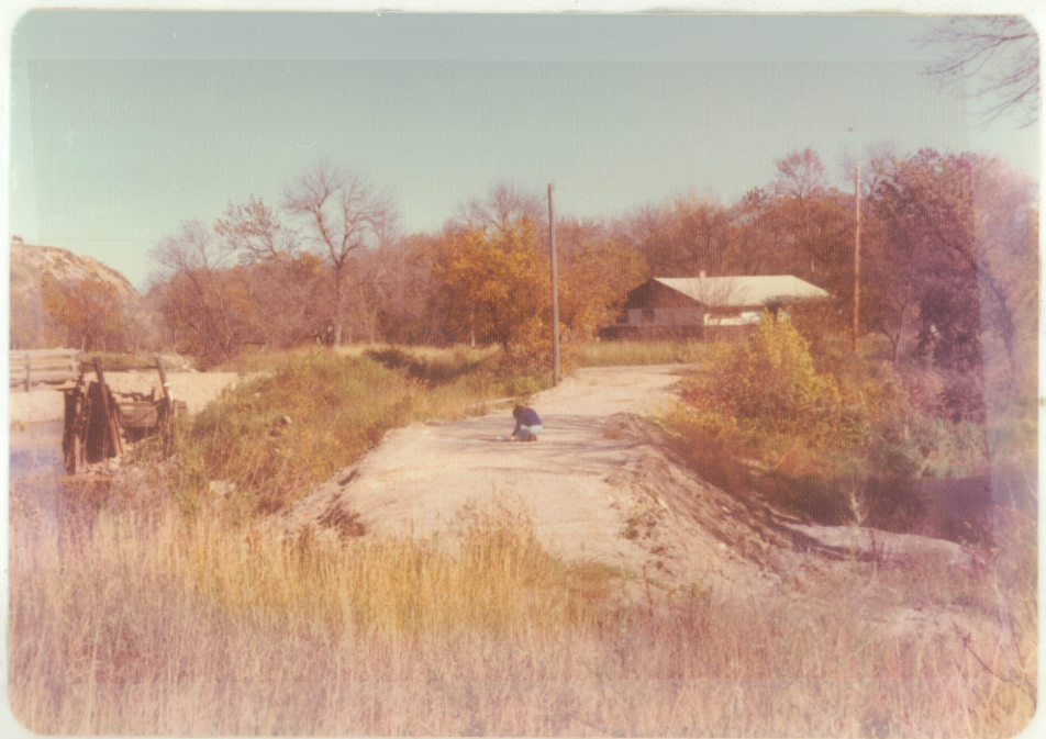
ESTEVAN DIVERSION DAM (B:8)
