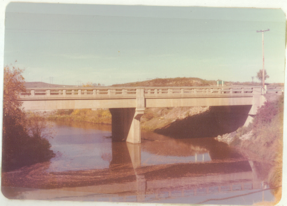
HIGHWAY BRIDGE (B:6)
