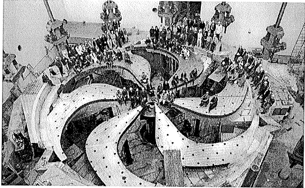
Figure 2.7: The completion of the lower magnet assembly of the TRIUMF cyclotron. The six main bending magnets are shaped to account for relativistic mass increase as particles accelerate to hundreds of MeV. Photograph taken in 1972 [24].
