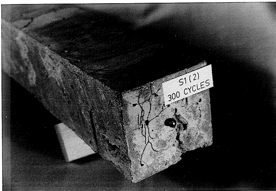
Figure 4.10: Photograph of Specimen S1(2) After 300 Cycles of Freeze-Thaw Showing Aggregate Related Distress.
