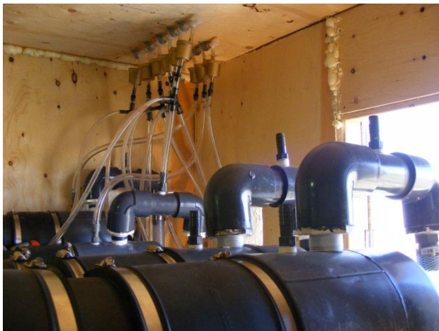
End of pipes with pipe rings inside of the pumps rubber clamps and pipe outlet
