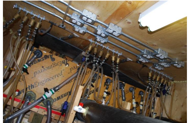
Air venting lines
