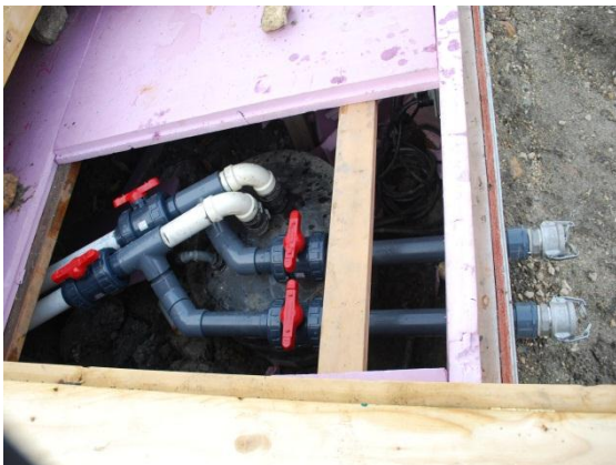
Leachate feeding lines and evacuating valves
