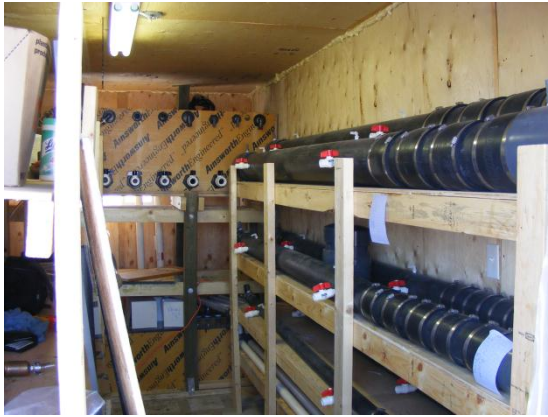
Pipes within the shelves
