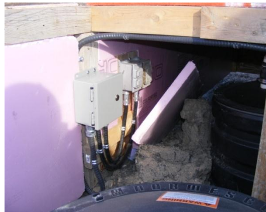
Electrical pump and heater wiring connection
