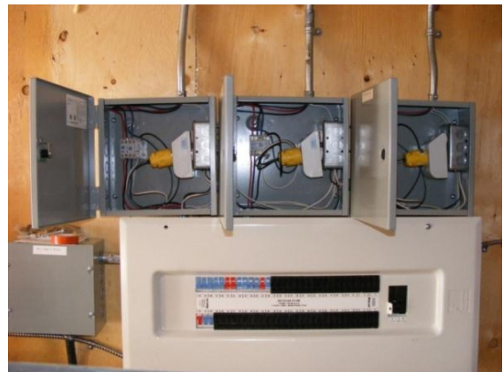
Electrical panel with 3 separate circuits
