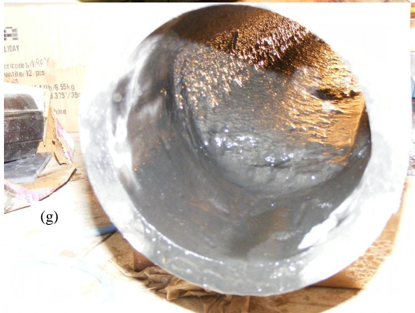
Figure (f) shows the clog accumulated within the pipe 7a after the pumps were turned off. Figure (g) shows the performance of the tool shown in (d) after clog was removed from the pipe outlet.
