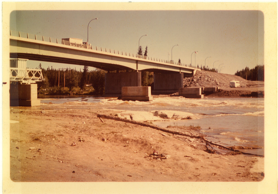
PHOTOGRAPH II-7 Thompson Bridge Overfall
