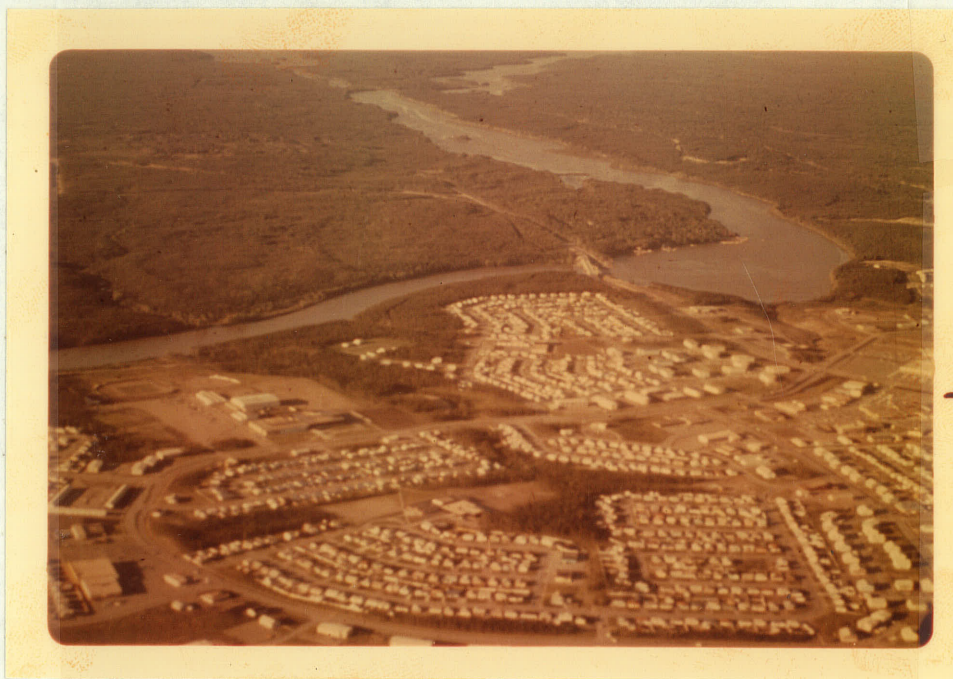
PHOTOGRAPH B1-5 Reach Near Thompson Bridge
