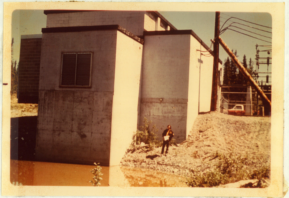
PHOTOGRAPH B1-1 Thompson Waterworks Pumphouse
