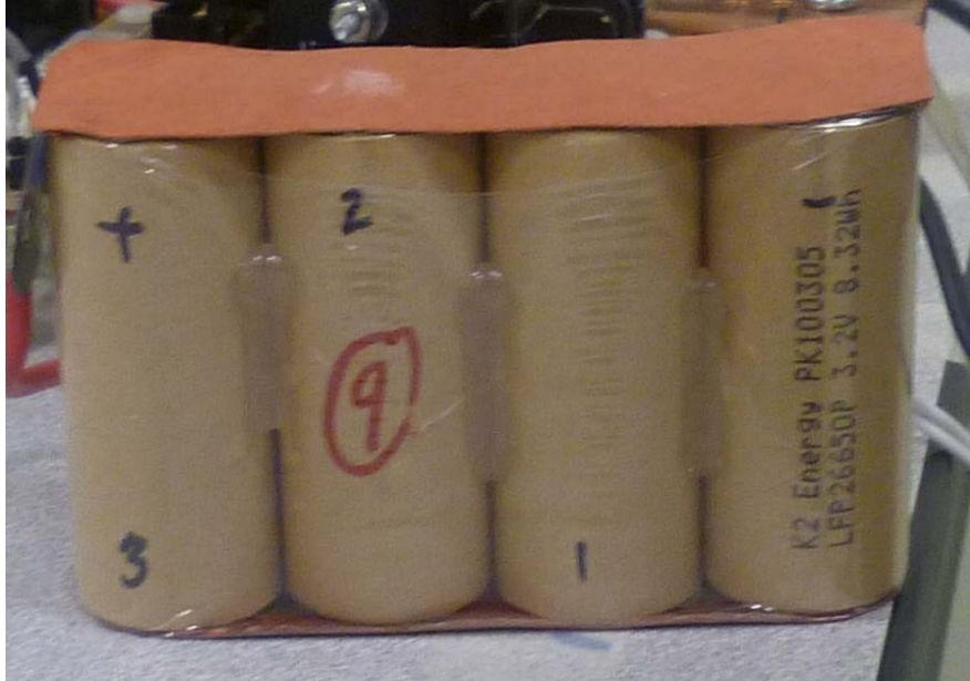
Figure 4-6: K2 Energy Constructed battery pack.
