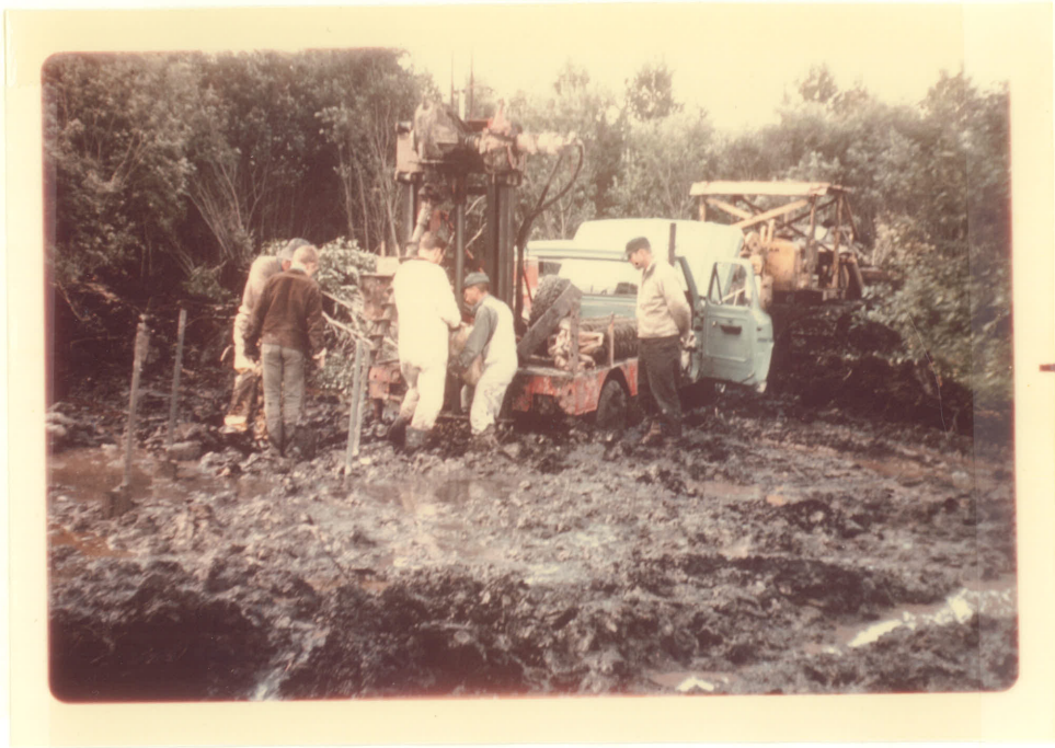
Fig. 9A Installation of piezometers in central discharge area.
