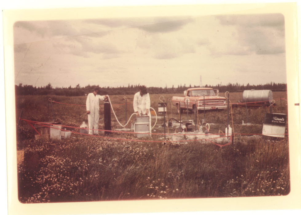
Fig. 13A Injection of tritium tracer at injection site No. 1.
