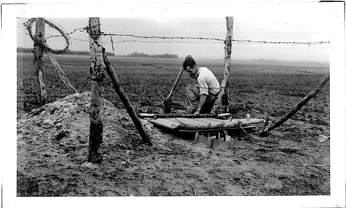
Figure No. 28 - View of leachate catchment site in a summerfallow field S.W. 34-14-12 showing tin enclosures at soil surface to prevent runoff.
