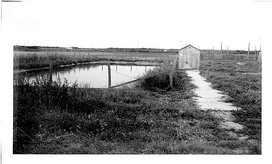
Figure No. 21 - View of Langruth dugout and reservoir, showing pump house enclosing pressure system. Water obtained from top to the left of pump house door contains nitrates. Water dipped from dugout showed absence of nitrate.
