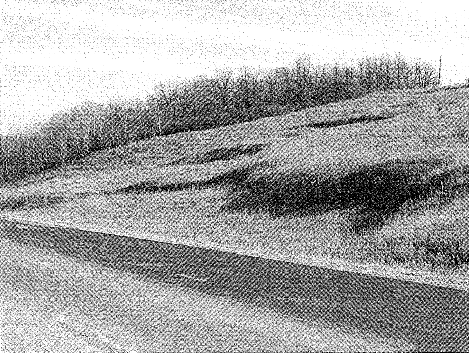
Figure 4.4 – Site 2 of PR259 and Assiniboine River, scattered retrogressive shallow shear failures
