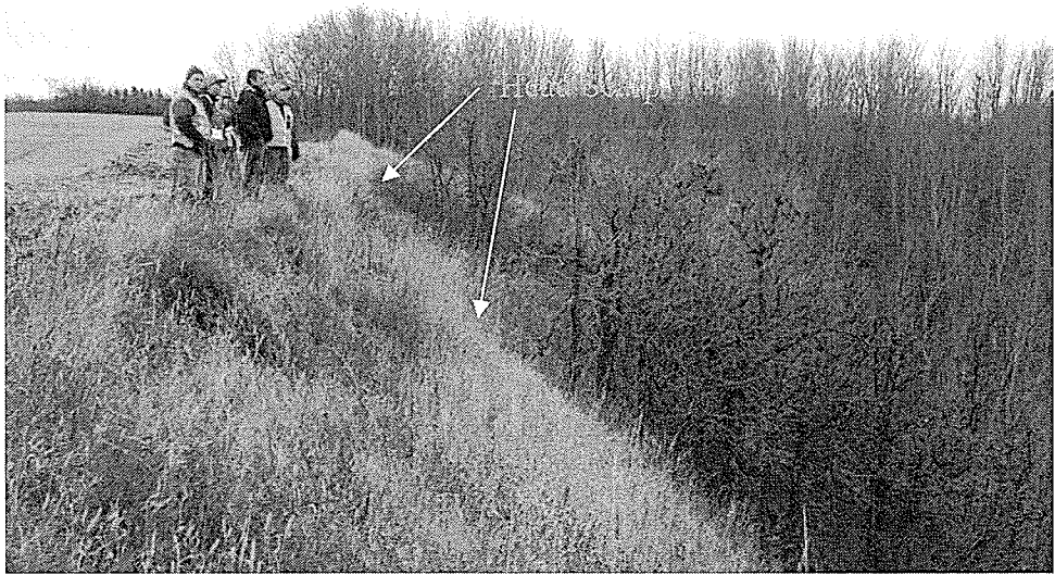
Figure 4.19 – PTH83 and Shell River, upper scarp of the larger mass movement
