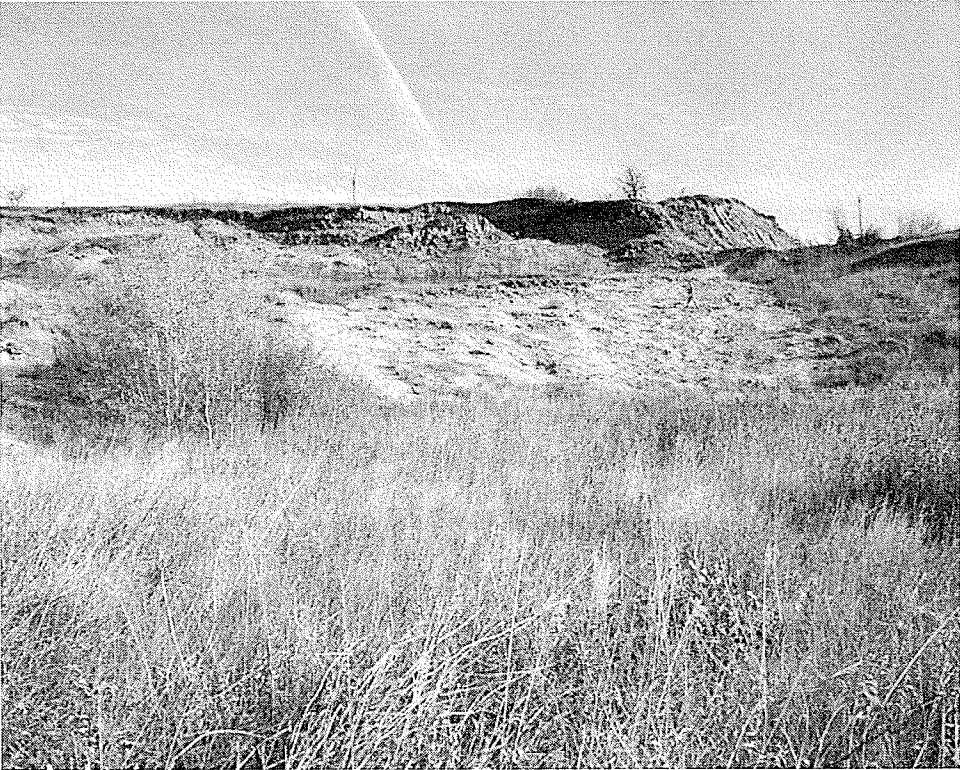
Figure 4.5 – Site 3 of PR259 and Assiniboine River, large scale failure
