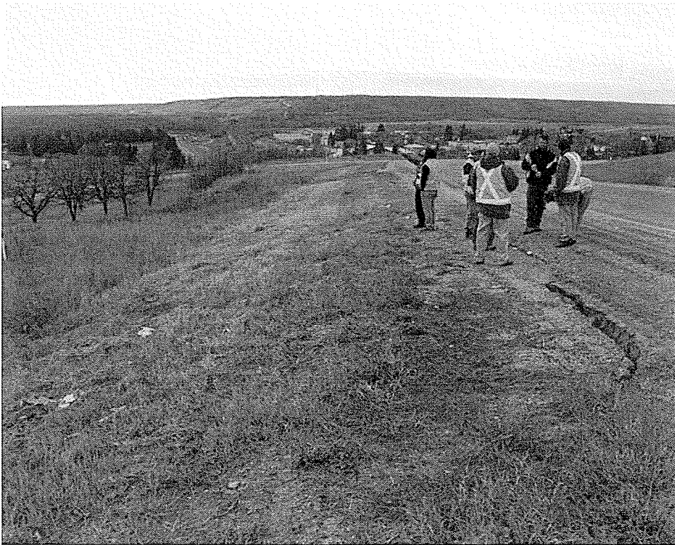
Figure 4.10 – Site 1 of PTH41 and Assiniboine River, large tension crack near roadway
