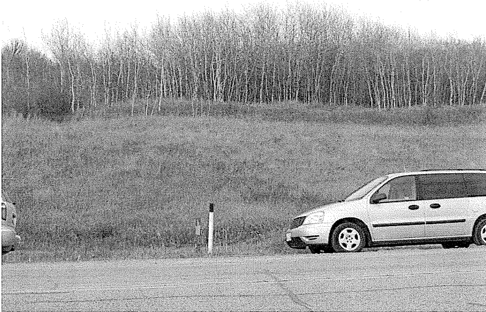
Figure 4.9 – Site 1 of PTH41 and Assiniboine River, retrogressive failure located on upper embankment
