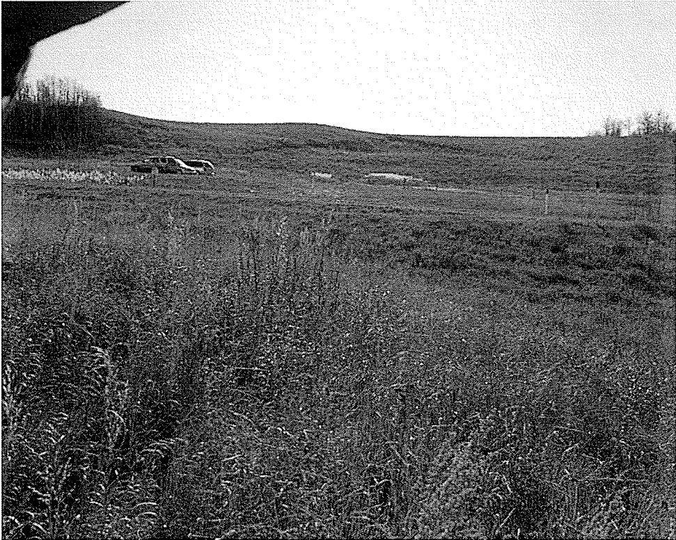
Figure 4.14 – PR478 and Assiniboine River, head scarp at top of upper slope
