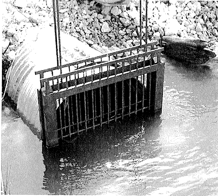
Figure 3.6: The photo shows the west-side of the culvert that runs under the road separating Mid-Blind Channel from the main area of the marsh. The removable grate was put in place for the spring of 2002 to prevent large fish from accessing Mid-Blind Channel. The pond is located on the opposite side of the road from where the photo was taken.
