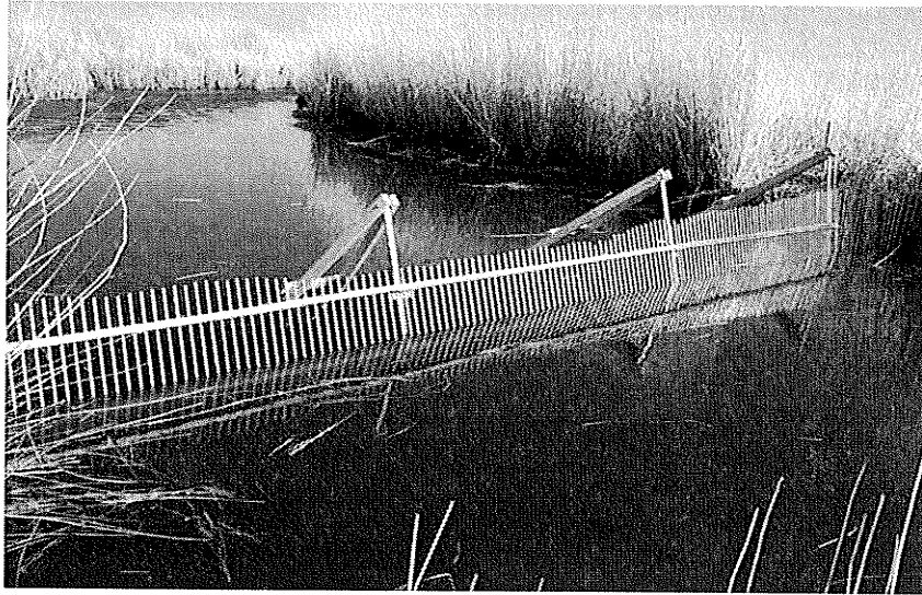
Figure 3.7a: The photo above shows the conduit fence on Cram Creek that was erected to prevent large fish from accessing Section 5 Bay during the summer of 2002 (Figure 3.5). The picture was taken shortly after construction, soon after wire mesh was added to the top of the fence to extend its height. The channel width was 10.7 cm.
