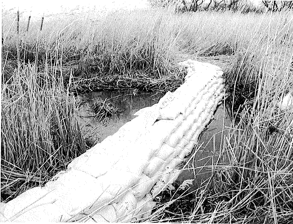
Figure 3.10: Sandbag dike isolating South Pitblado's Channel from the main area of Delta Marsh during the summer of 2002. A similar dike was also erected to isolate Mad Woman Bay.
