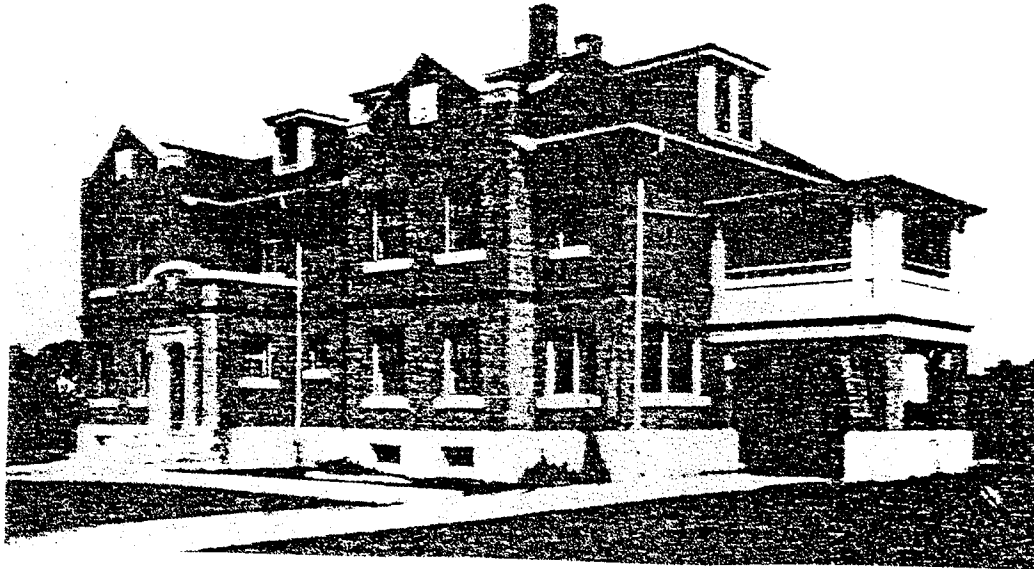
FIGURE 22 : Principal's Residence, Manitoba Agricultural College, St. Vital site (1913), Winnipeg
