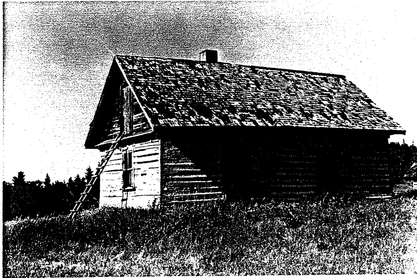
Plate 19b Ukrainian "early-transitional phase" residential types, -distinguishable from "traditional phase" examples by construction material and mode. (Top) the John Paulencu House near Lennard, Manitoba, an excellent Bukovynian example recently nominated for designation as a provincial heritage site, and; (bottom) the Wasyl Stelmach House, part of a superbly preserved Galician style farmstead set near Riverton, Manitoba. (Historic Resources Branch photos)
