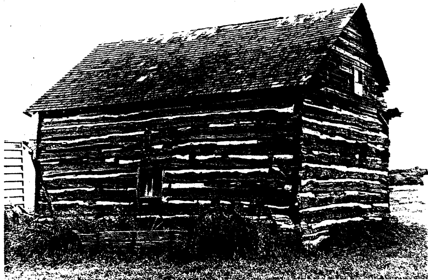
Plate 8c Abandoned farm structures: (above) 1882 shed, NE6-2-5W, near Morden, and; (below) ca.-1890 log granary, NW32-2-6W, near Thronhill. (Historic Resources Branch photos)
