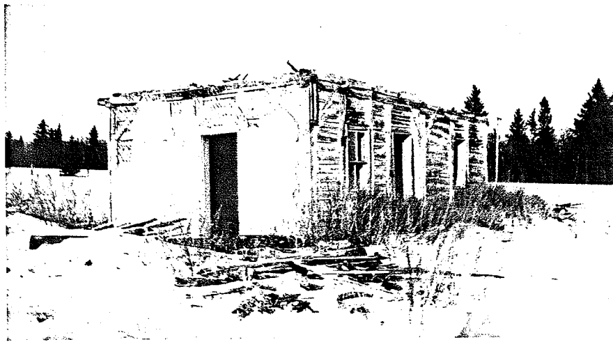
Plate 23 Former J. Andrusiak residence, NE22-20-2W. This log farmhouse is only one of a number of vintage farm structures located along PTH #7 which have recently been demolished.
