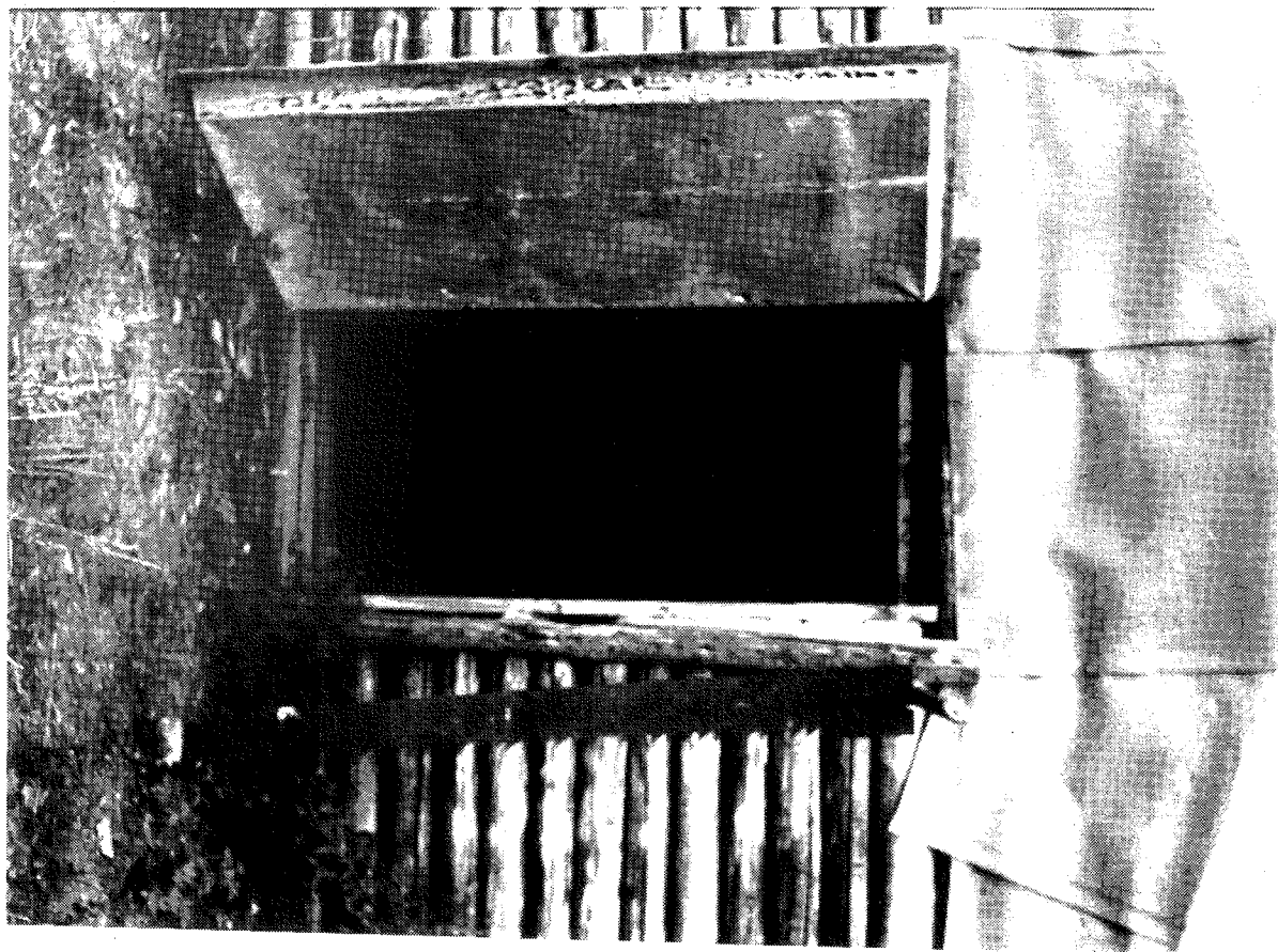
Fig. II.48 site 113 - ice house door showing thickness of insulation.
