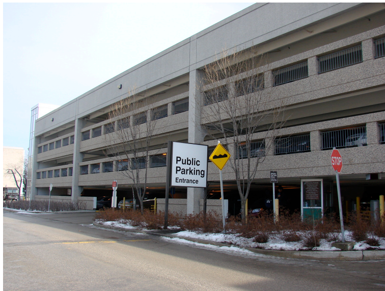
Figure 6: View of Public Parking Lot/Parkade
