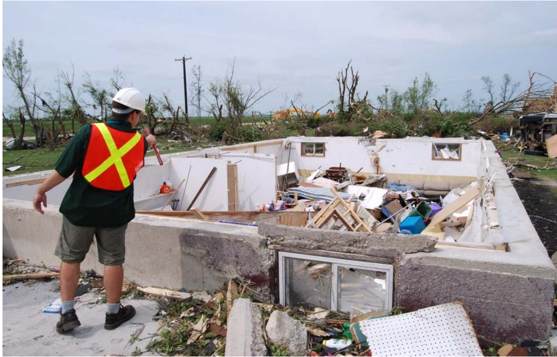
Figure 1.13: Storm damage survey picture taken on 23 June 2007 in Elie, MB showing foundation remaining after house was lifted and led to disintegrate in mid-air (PASPC Image Archive, 2007).
