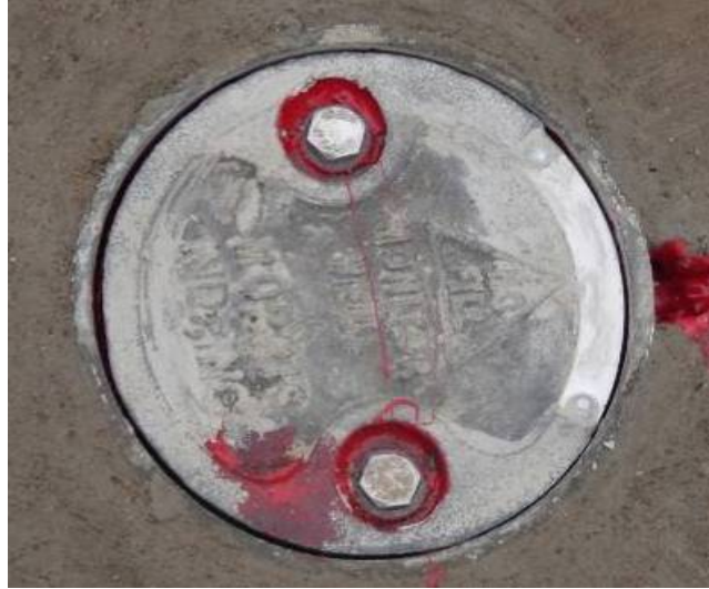
Figure A-44 MDD assembly fully installed at PTH11.
