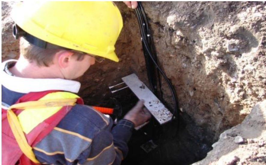
Figure A-10 Using a pilot tool to install WCR probe at PTH11.
