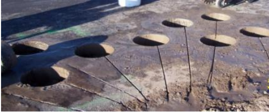
Figure A-46 Grooves for sensor wires were cut diagonally to the edge of pavement (PTH11).
