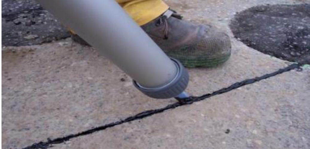
Figure A-47 Sealing groove after wires were inserted (PR304).
