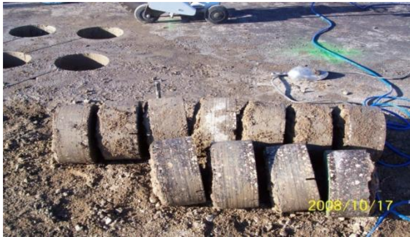
Figure A-8 AC cores extracted at the test site of PTH11.
