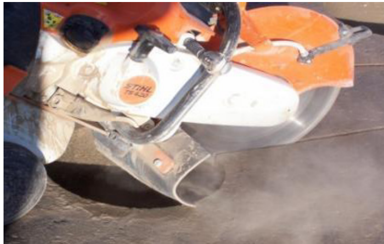
Figure A-45 Cutting a groove in AC layer for a sensor wire (PTH11).
