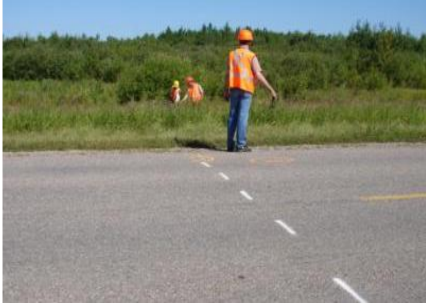
Figure A-4 Test section at PR304.
