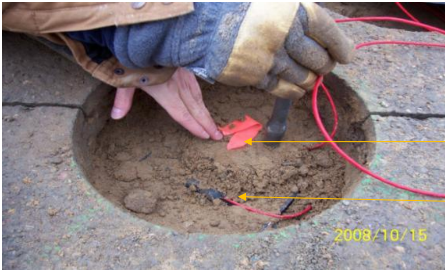
Figure A-29 Horizontal and vertical ASGs were installed together in base layer of PR304.
