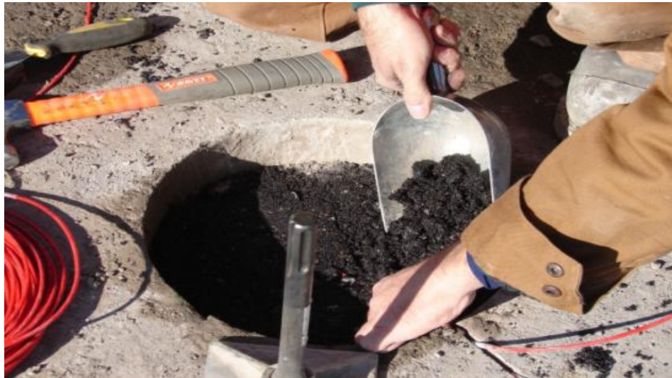
Figure A-27 Installing horizontal ASG at PTH11.
