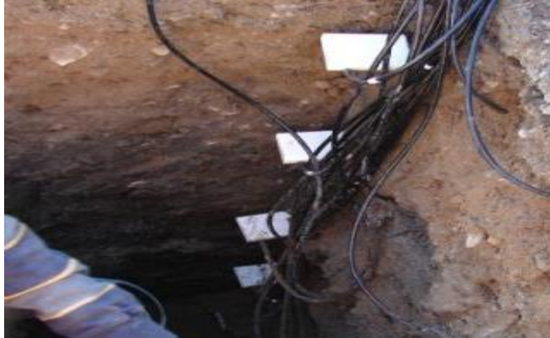
Figure A-11 Five WCR probes were installed at PTH11.
