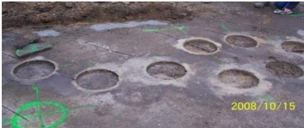
Figure A-24 Core hole arrangement for strain gauges at PR304.
