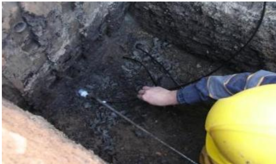
Figure A-16 Inserting a FTC into a drilled hole with sensor insertion tool at PTH11.
