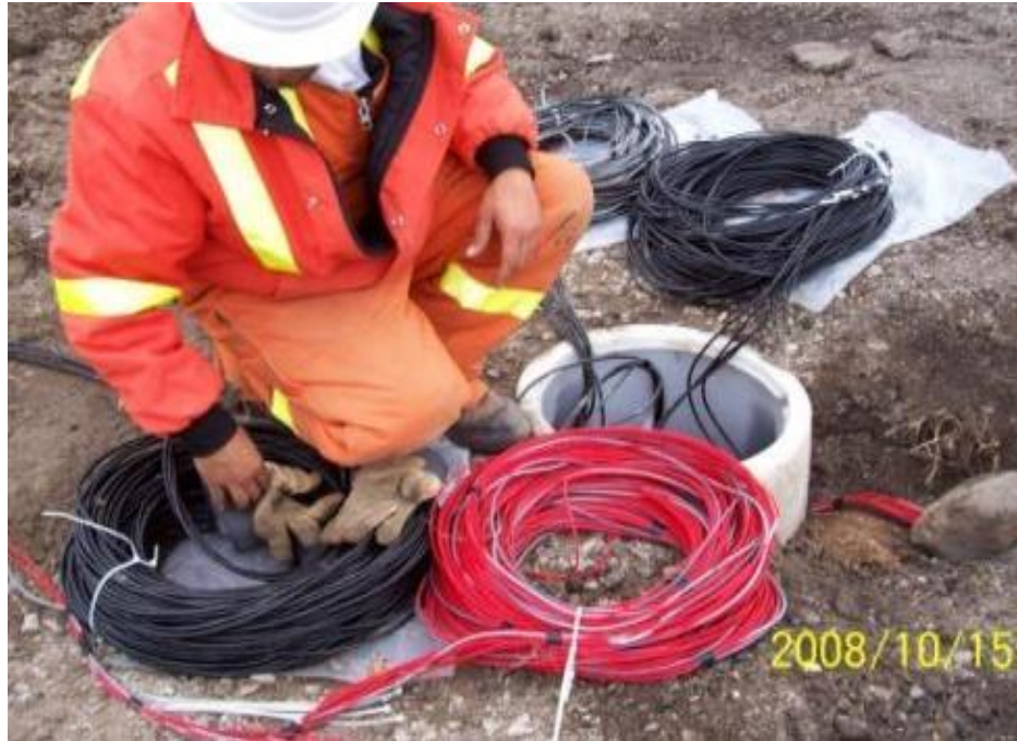
Figure A-48 Splicing pit.
