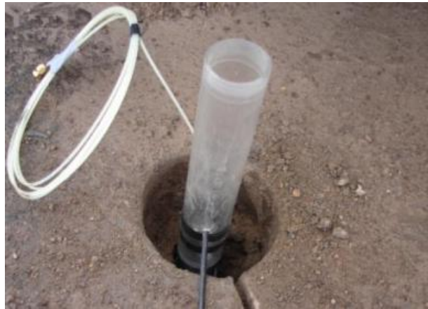
Figure A-39 Precisely setting the MDD elevation with a pinned setting tube.
