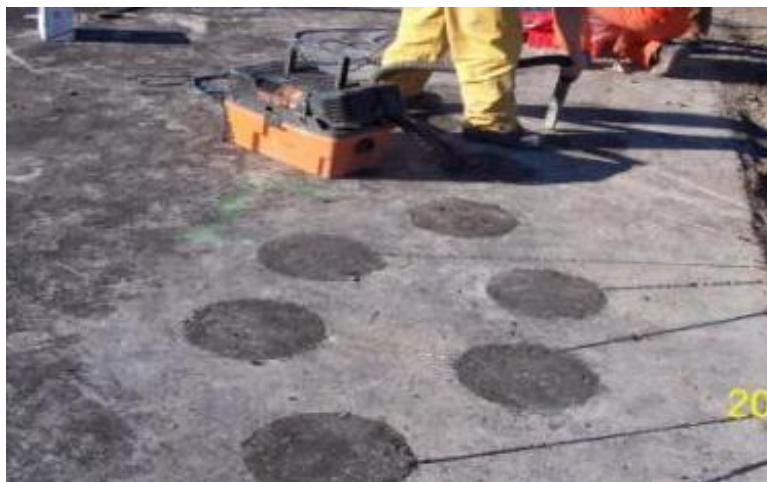
Figure A-31 Strain gauge holes backfilled with compacted cold mix at PTH11.
