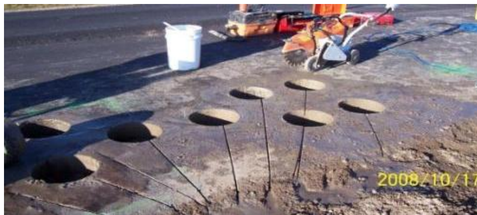
Figure A-25 Core holes with saw cut grooves for wire leads at PTH11.
