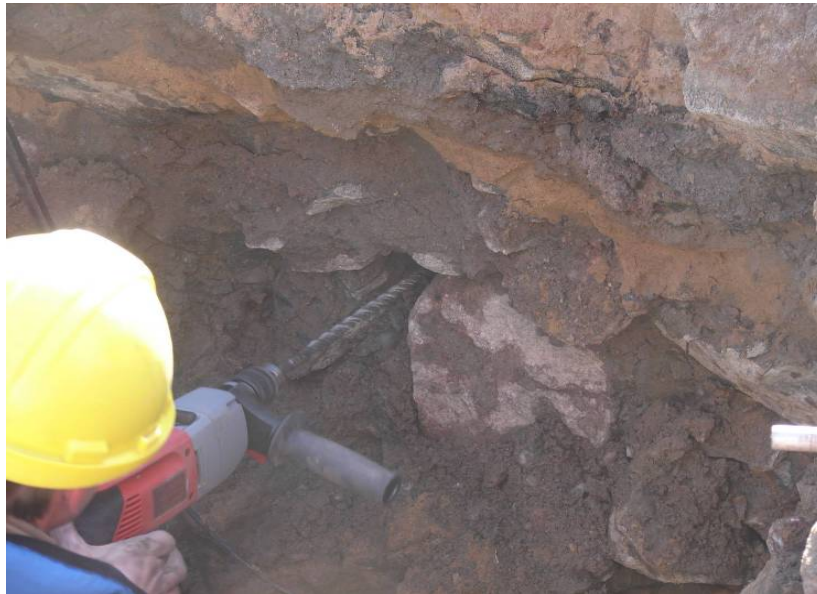
Figure A-6 500 mm rock fill visible in an excavation in the shoulder of PR304.
