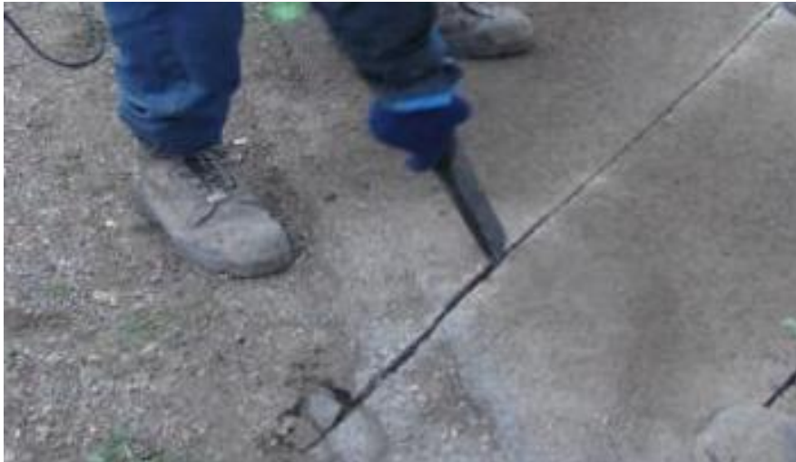
Figure A-49 Cleaning wire grooves (PR304).
