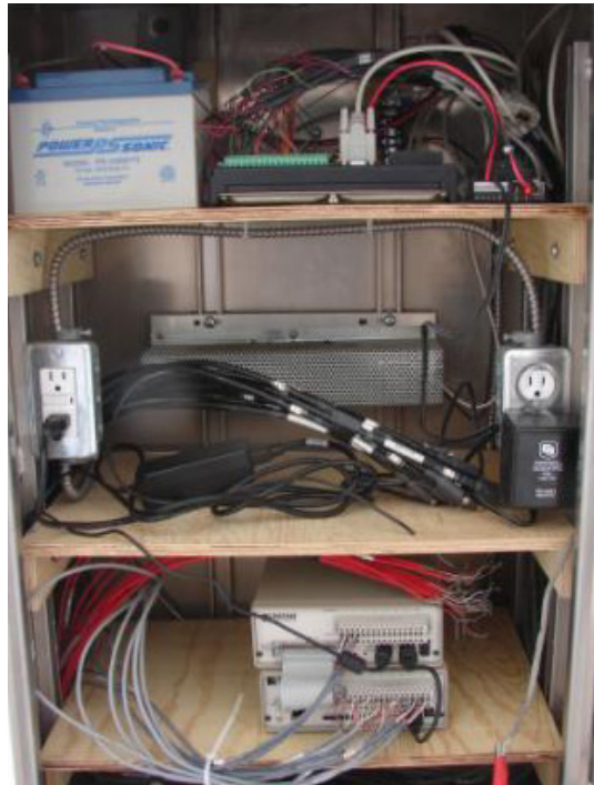
Figure A-54 Cabinet and data acquisition system at PTH11.
