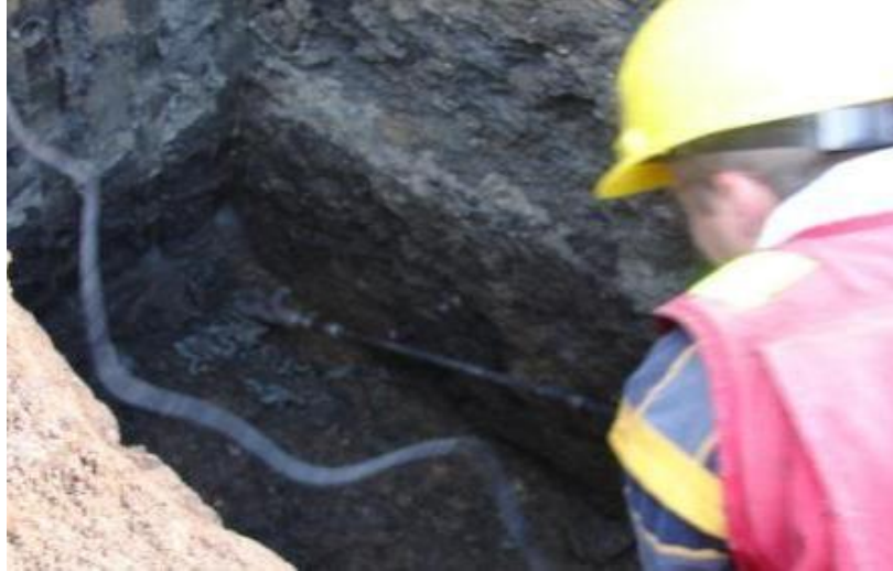
Figure A-15 Drilling a hole for installing an FTC with 28 mm diameter auger at PTH11.
