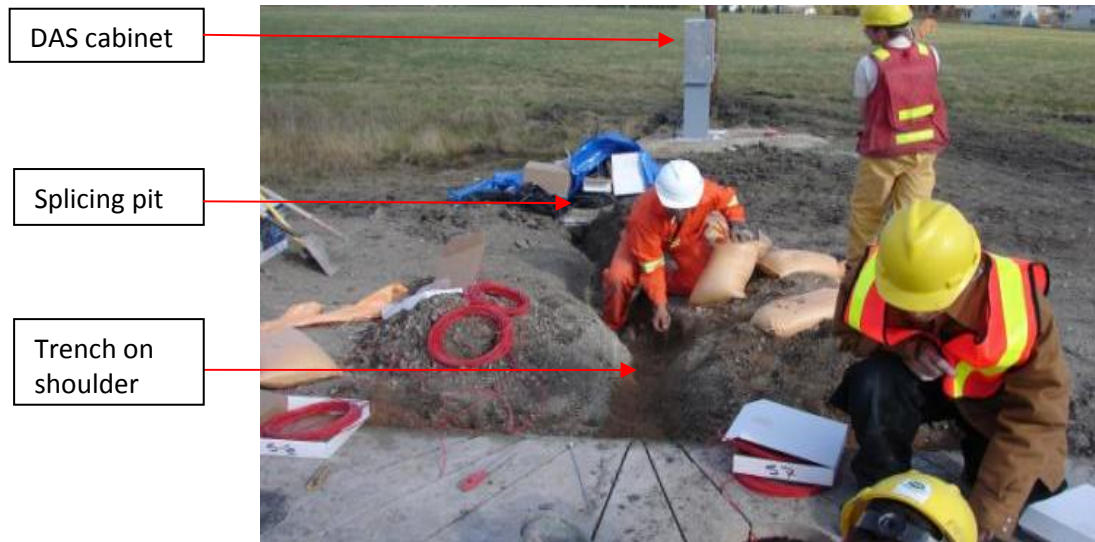
Figure A-49 Wiring was routed from roadbed via trench and splicing pit to DAS cabinet.
