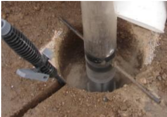
Figure A-41 Backfilling the annular space around the MDD.
