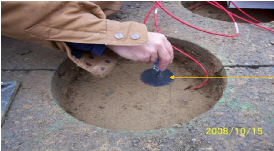
Figure A-29 Installing vertical ASG into granular base layer of PR304.
