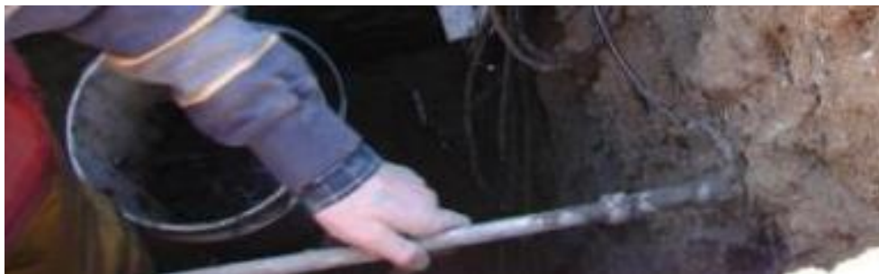
Figure A-17 Backfilling the hole using tamping dowel after inserting a FTC.
