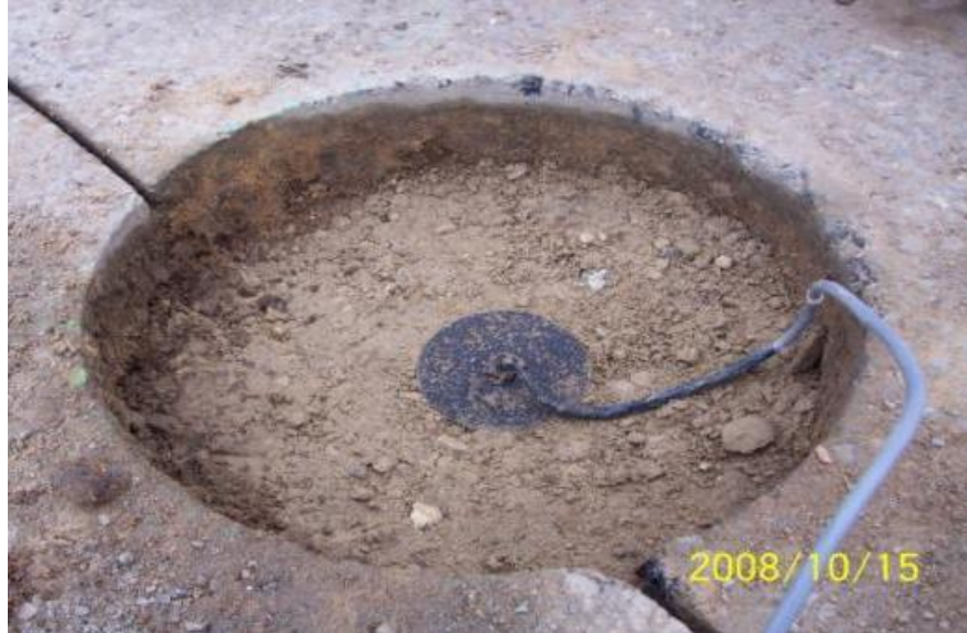
Figure A-33 A SCG installed into granular base layer of PR304.
