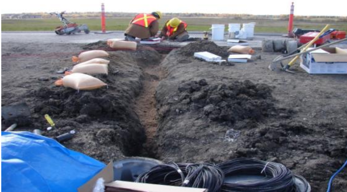
Figure A-51 Trench to splicing pit.
