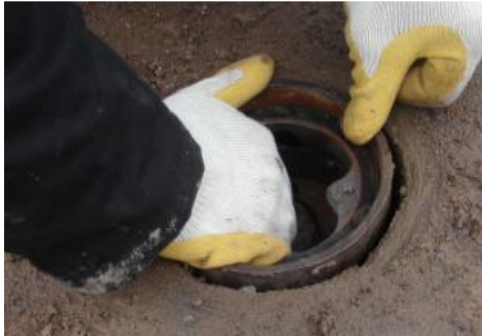
Figure A-42 Inserting MDD road box into AC layer.
