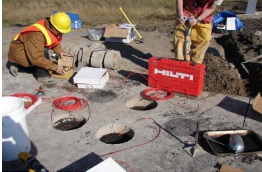
Figure A-28 Strain gauges installation at PTH11.
