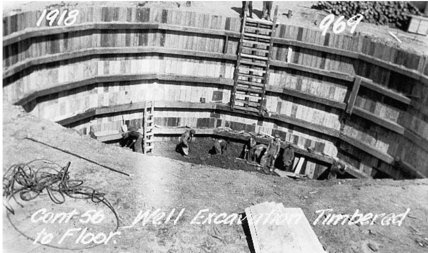
Figure 8.11.1 Shoring for surge tank excavation (GWWD No. 969)
