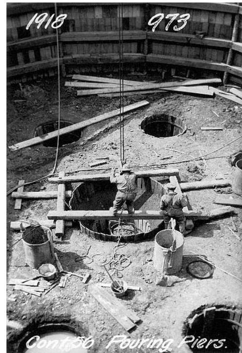
Figure 8.11.2 Caisson construction (GWWD No. 973)
