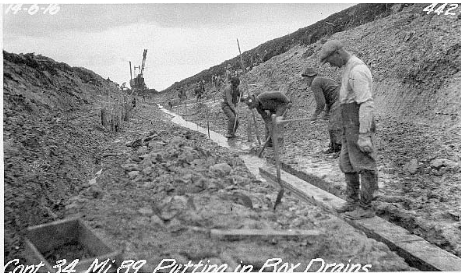
Figure 8.7.2.1. Box drain installation (GWWD No. 442)
