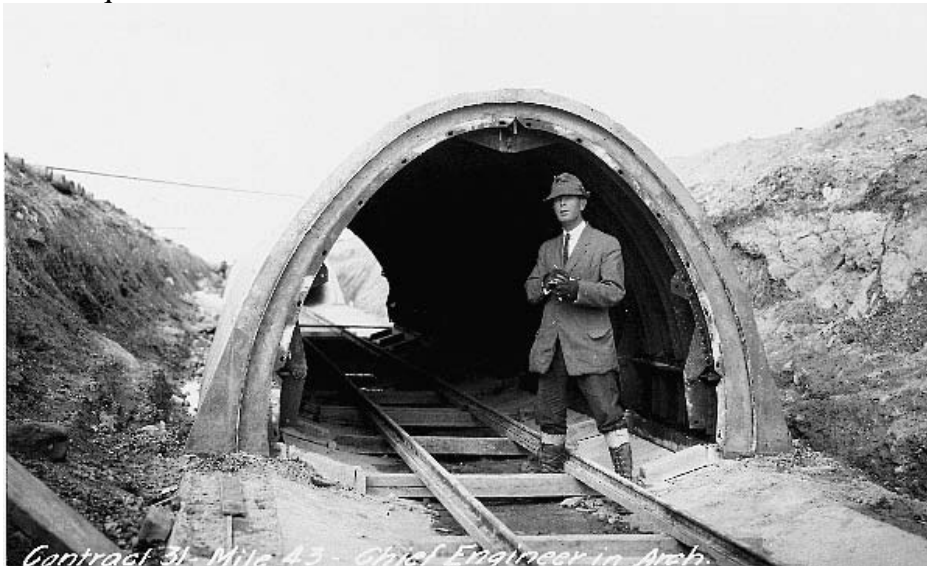
Figure 7.3.2. Chief Engineer W.G. Chace at a typical arch section on an invert (GWWD No. 264)
