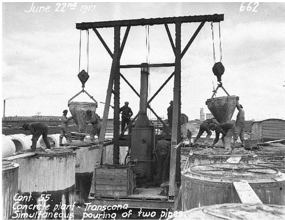
Figure 8.9.1. Lock Joint concrete pipe manufacturing (GWWD No. 662)
