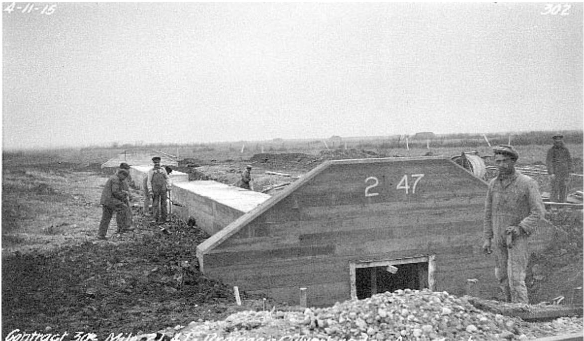
Figure 7.11.1. Cross drainage culvert with depressed middle section (GWWD No. 302)
