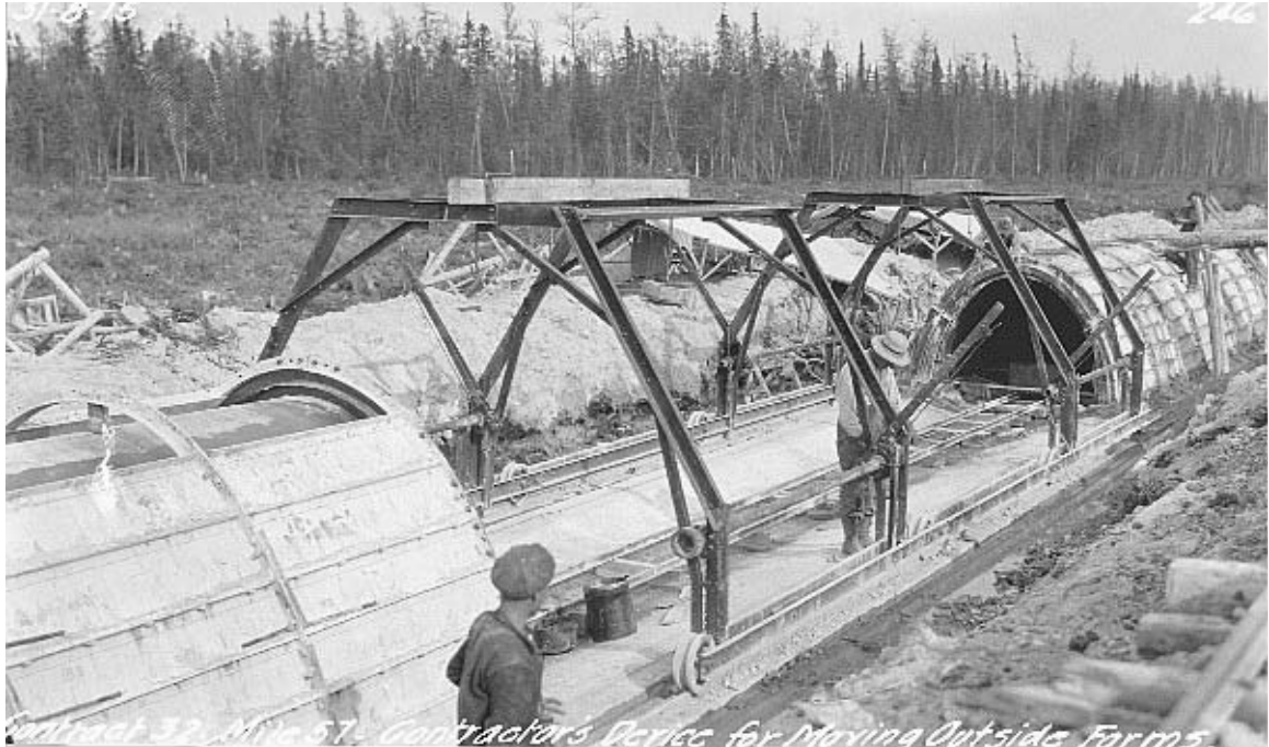
Figure 8.7.5.2 Traveller system for moving arch forms along conduit (GWWD No. 246)
