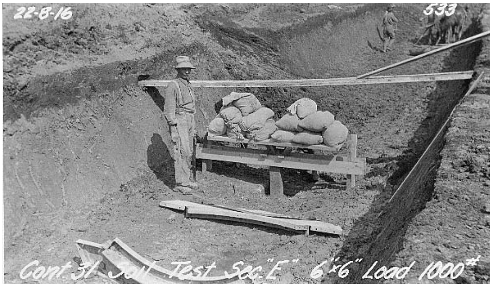
Figure 8.5.1.1. Onsite soil bearing test (GWWD No. 533)
