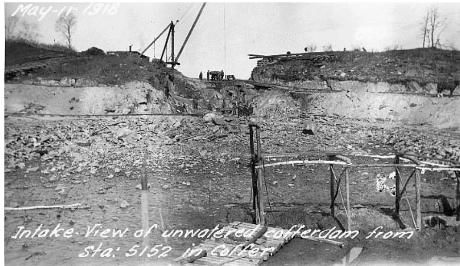
Figure 8.3.3. Intake cofferdam unwatered (GWWD No. 880)
