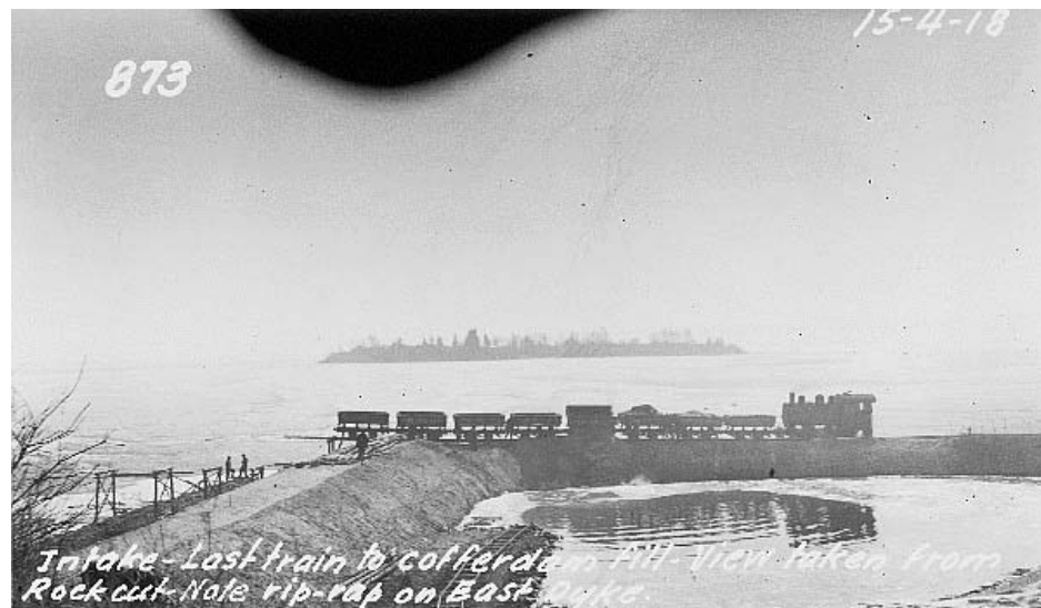
Figure 8.3.2. Intake cofferdam before dewatering (GWWD No. 873)
