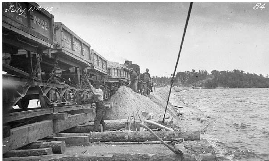
Figure 7.12.1. Construction of the Falcon River Dike (GWWD No. 84)
