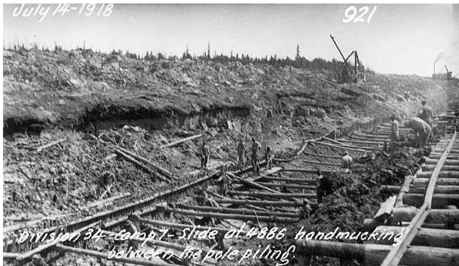
Figure 8.7.1.3. Remedial work on side-slope failure zone (GWWD No. 921)
