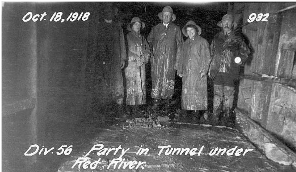
Figure 8.10.1. Visitors on tour in the Red River crossing tunnel (GWWD No. 932)
