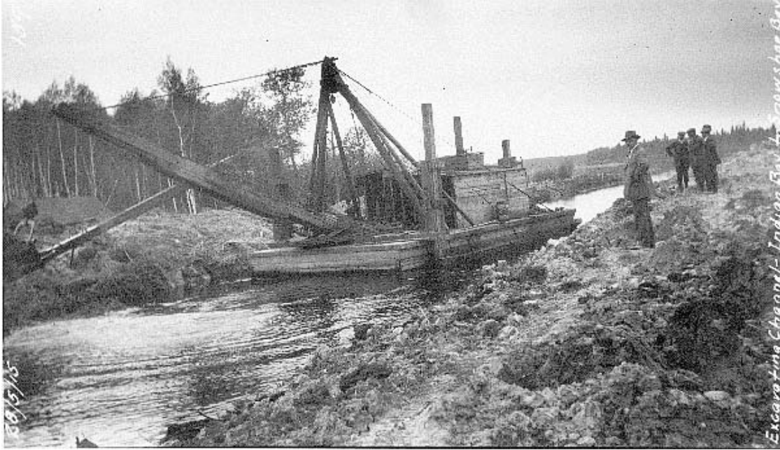
Figure 8.2.1. Channel excavation from Indian Bay to Snowshoe Bay (GWWD No. 159)
