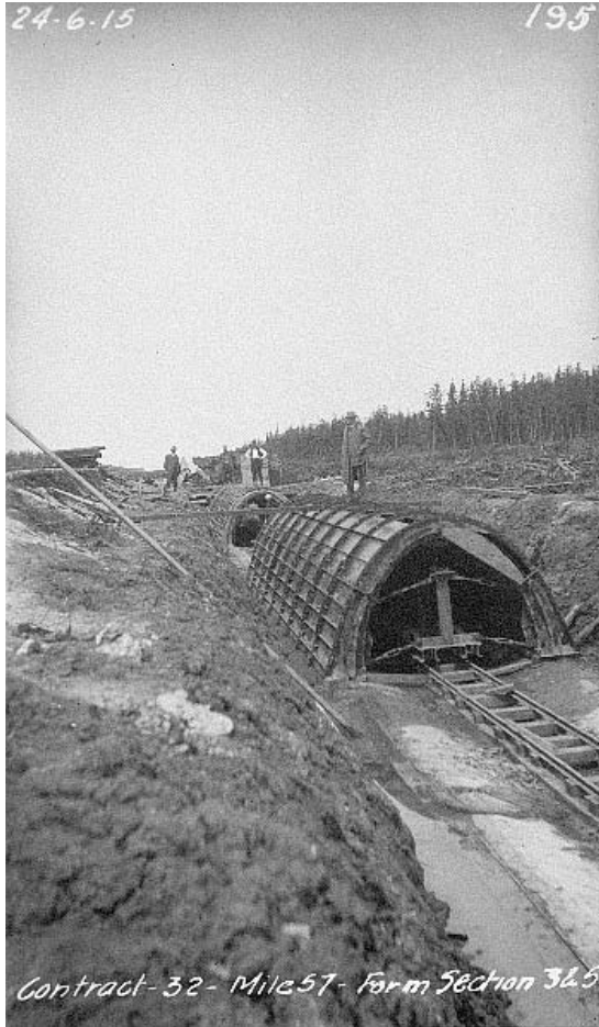
Figure 8.7.5.1 Blaw steel arch forms in position (GWWD No. 195)
