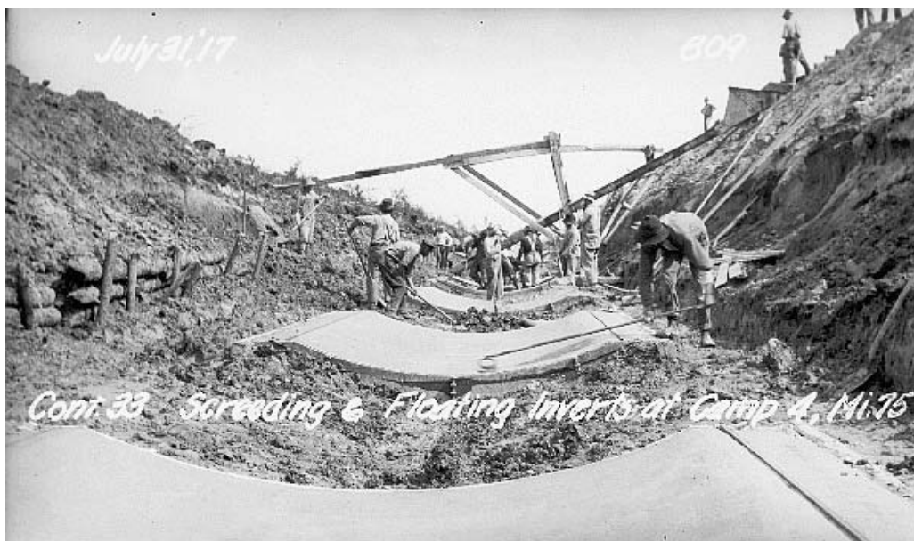
Figure 8.7.4.1. Placing invert concrete (GWWD No. 809)
