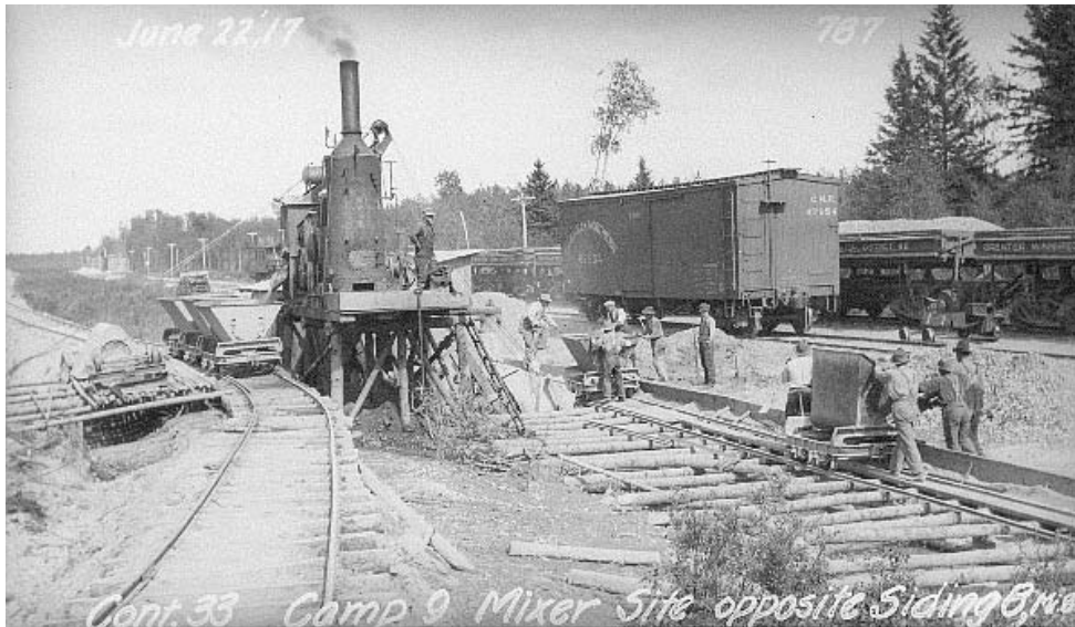
Figure 8.7.3.1. Concrete mixing and transport system, Winnipeg Aqueduct Construction (GWWD No. 787)
