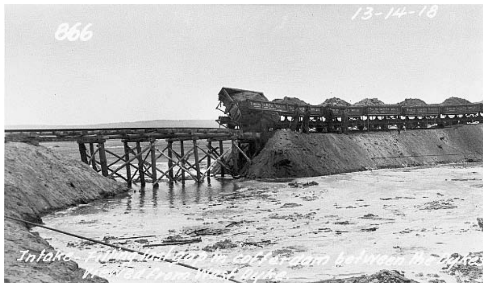
Figure 8.3.1. Intake cofferdam construction – closure (GWWD No. 866)
