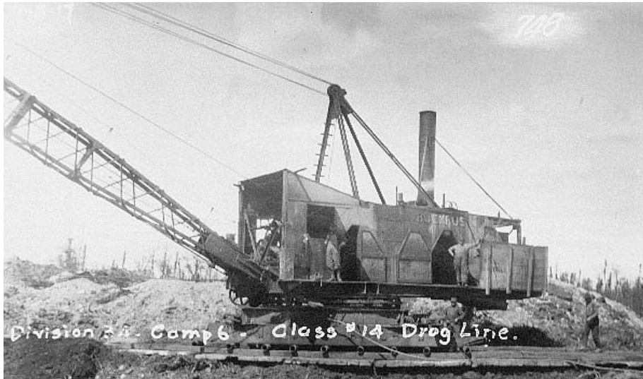
Figure 8.7.1.2. Dragline with support and propulsion system (GWWD No. 748)
