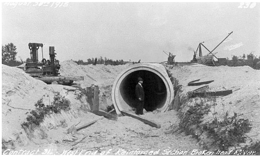
Figure 7.3.3. Circular pressure section west end of Brokenhead River slough (GWWD No.230)
