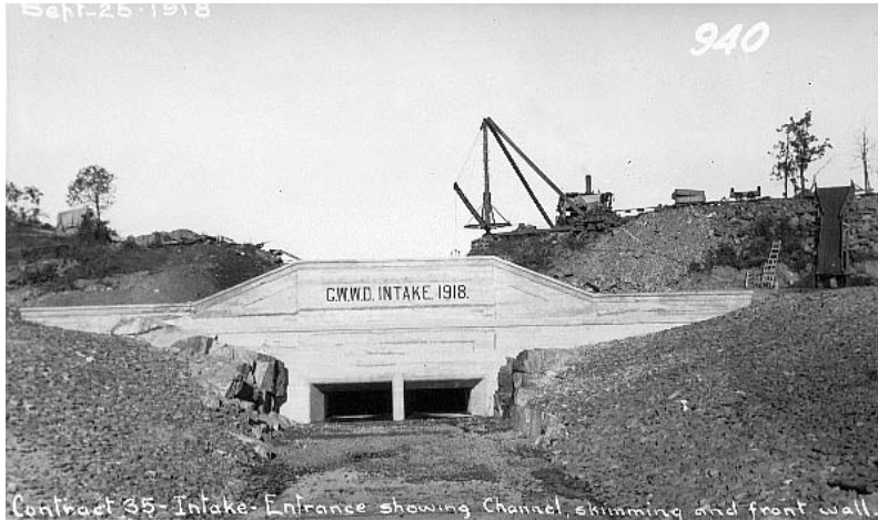
Figure 7.13.1. Intake structure before flooding (GWWD No. 940)
