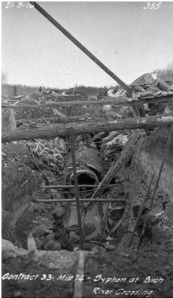
Figure 8.7.7.1. One end of an in-trench siphon construction (GWWD No. 355)
