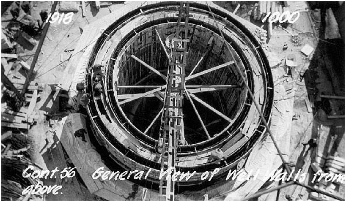
Figure 8.11.3. Forming system for the circular weir and containment wall (GWWD No. 1000)
