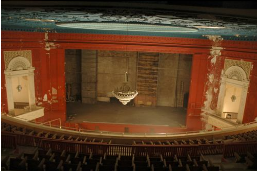
Figure 1-3: Interior view of the Theatre from Balcony, Courtesy: Number Ten Architectural Group.
