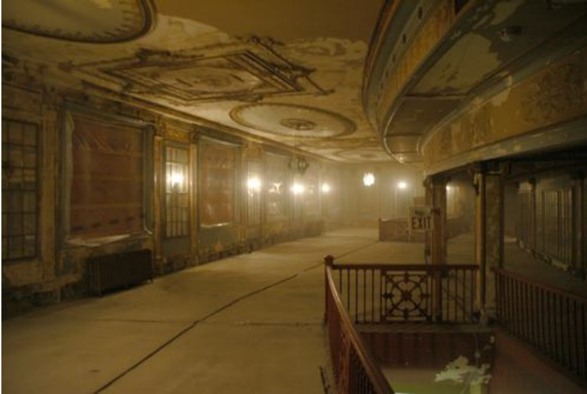
Figure 1-7: Interior View of Mezzanine. Courtesy: Number Ten Architectural group
