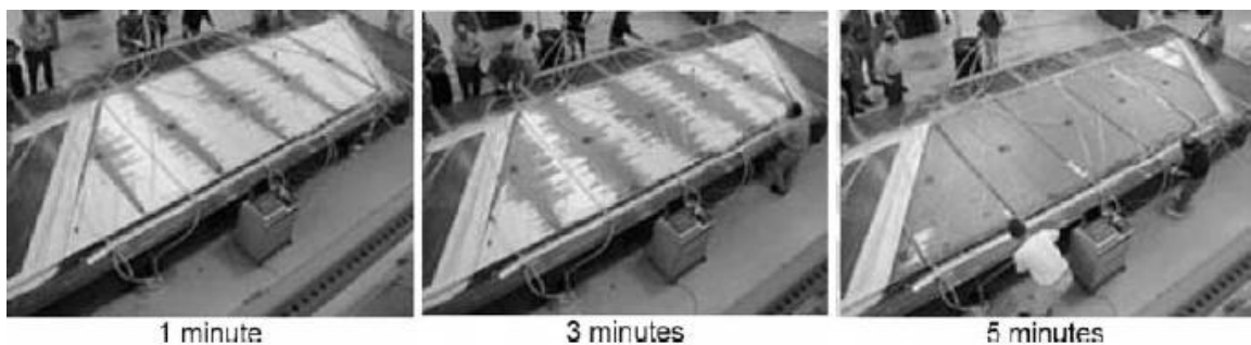
Figure 2.2: VARTM process on Tycor reinforced bridge deck (Telang et al., 2006)
