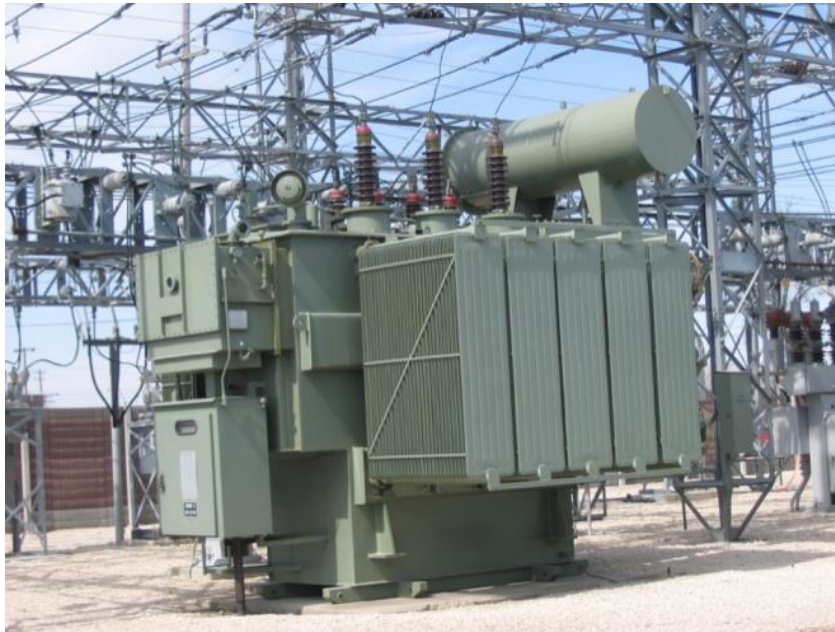
Figure. 1.1. A power transformer [4].
