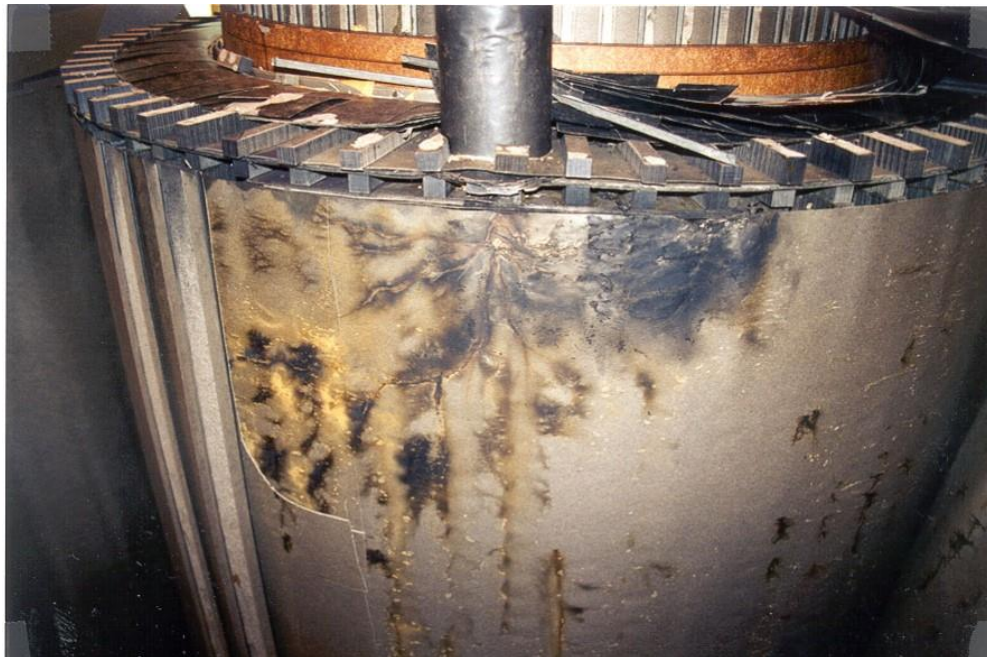
Figure 2.3. Converter transformer failure where evidence of partial discharge activity found on barrier surface between two windings [4].
