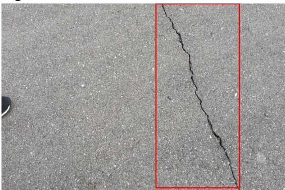
(a) Outside of EITC: pavement
