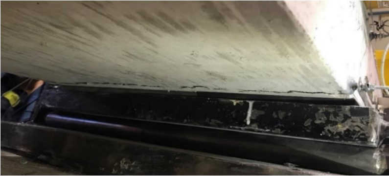
Figure 25 Crack under the slab close to support at the cantilever end of AR3
