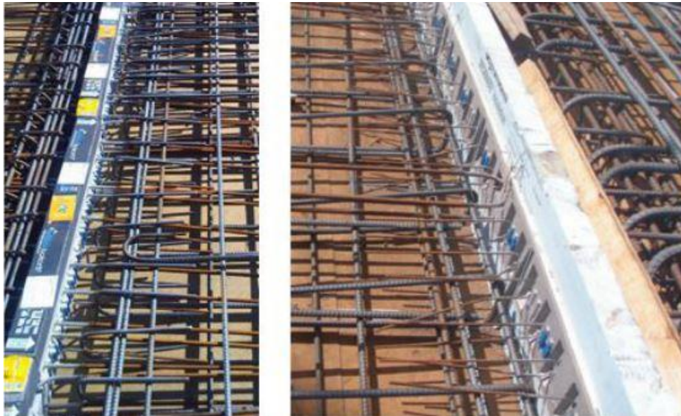
Figure 1 Schöck Isokorb® thermal break in concrete balcony (Chafik, 2015)
