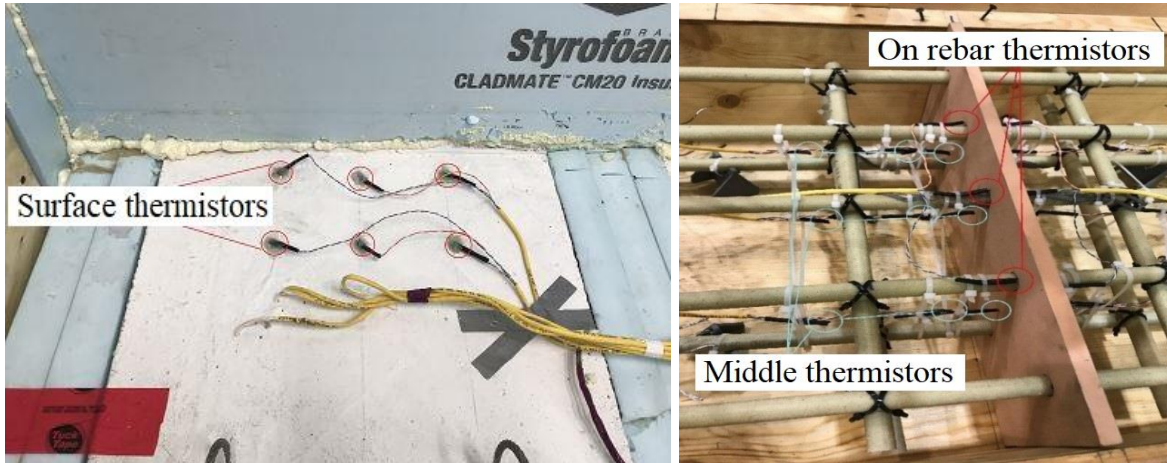
Figure 32 Top surface, on rebar, and middle thermistors
