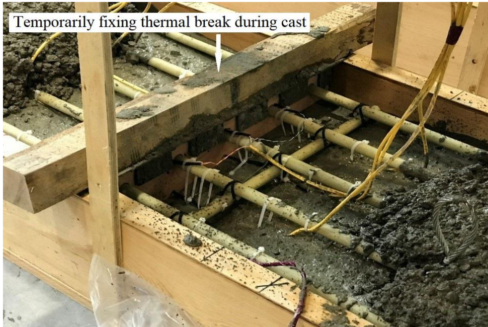
Figure 13 Temporary “fixer” for thermal break during cast
