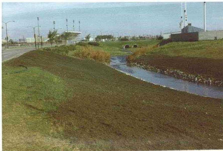
P22.2 Bank in P22.1 reshaped with a clay berm and riprap for erosion protection at the toe. Two horizontal trench drains were also installed.
