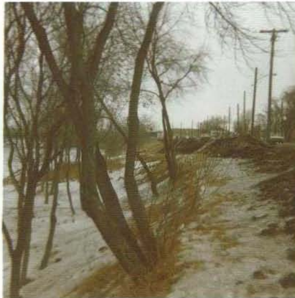
P4.2 Failure scarp of P4.1 with grass cover and small trees, Tache Avenue, 1971.
