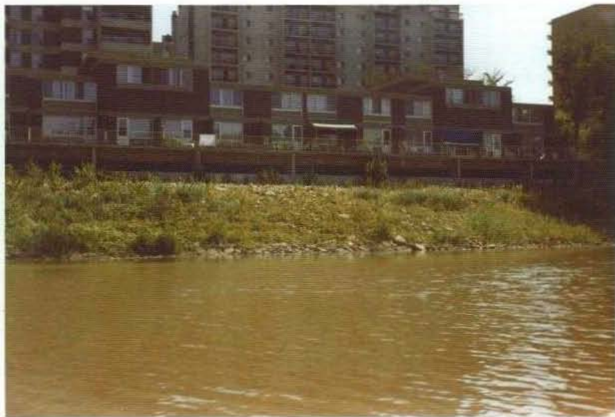
P9. Riprap protection of slope to above flood stage. Note failure of bank through riprap at right, Assiniboine River, 1972.
