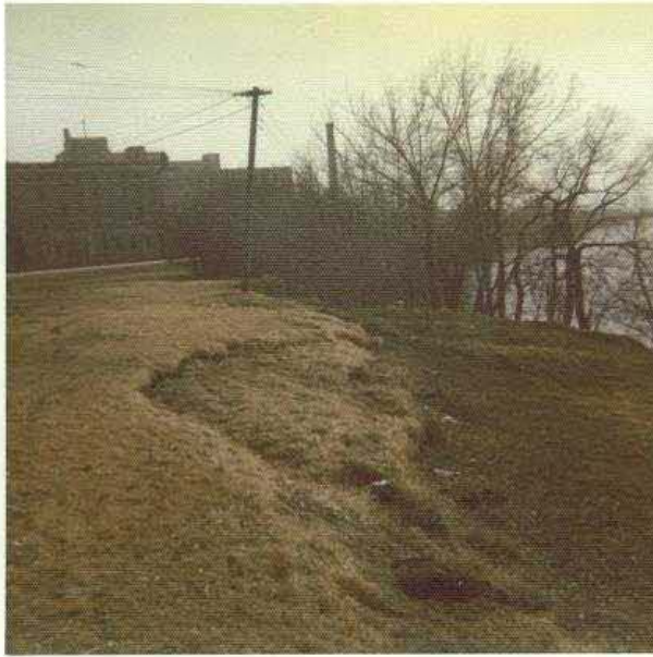
P5. Example of an older failure with fresh cracks and slumps appearing, Tache Avenue, 1971.
