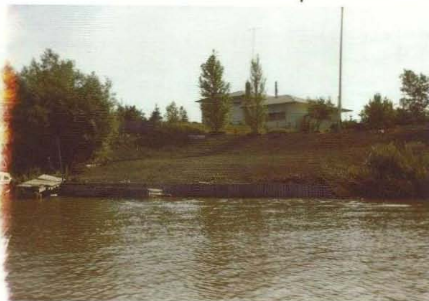
P8. Slope flattening to improve stability with a sheet piling retard for protection against erosion, Red River, 1972.
