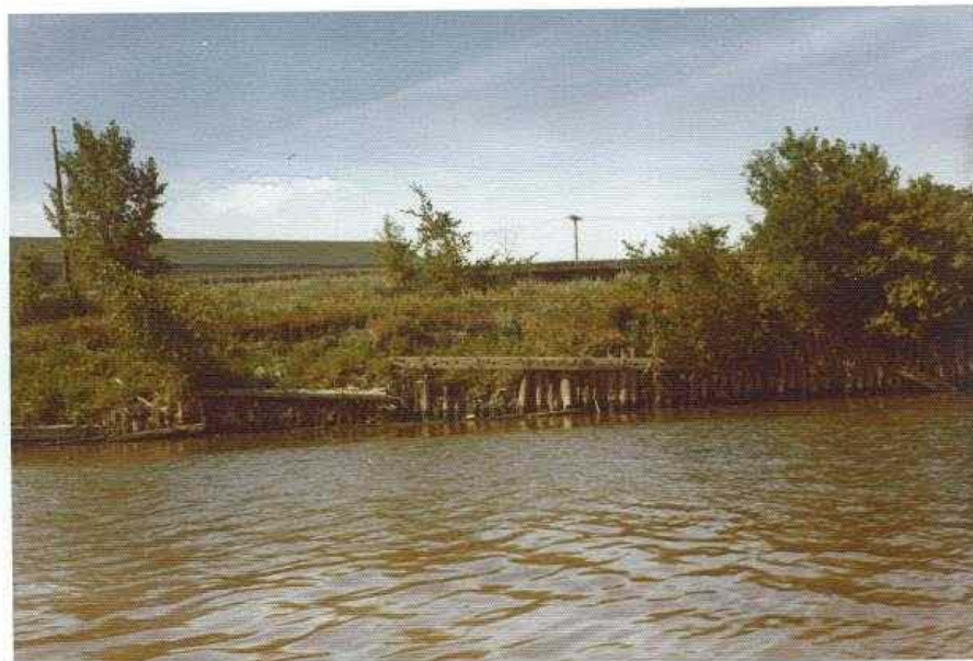
P17. Timber pile retard, piles closely spaced. Note condition of piles above summer water level and failure of bank behind damaged portion of retard. Red River, 1972.
