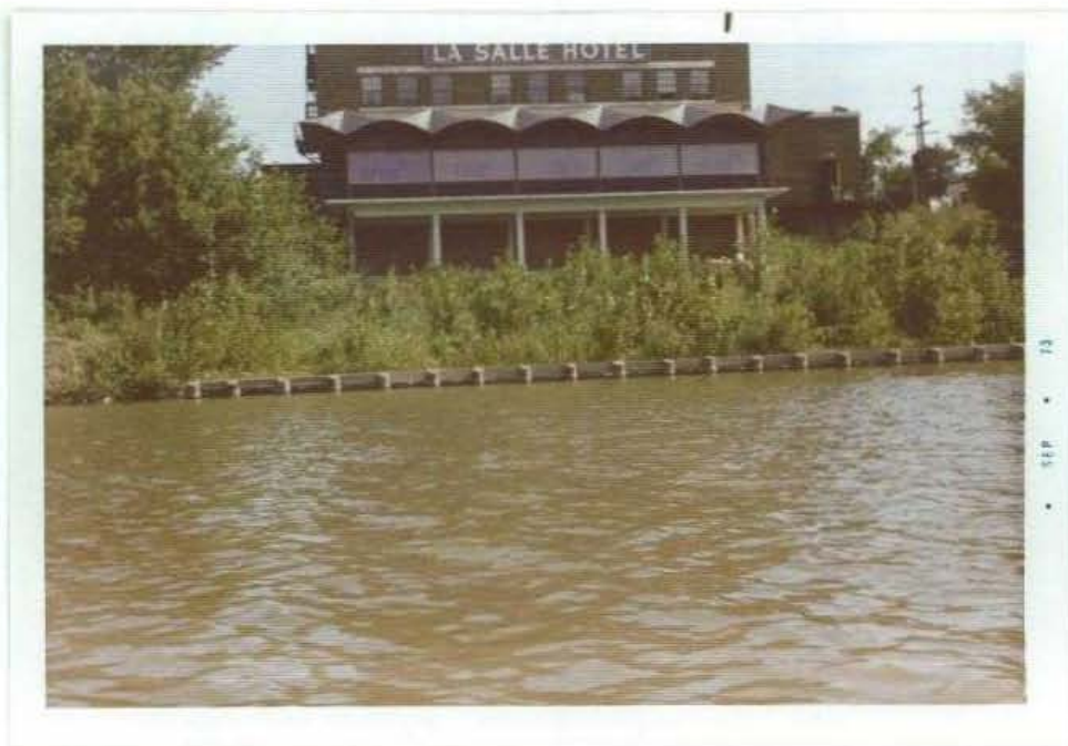
P21. Timber pile retard with horizontal planking. Note established growth of shrubs and small trees behind retard. Red River, 1972.
