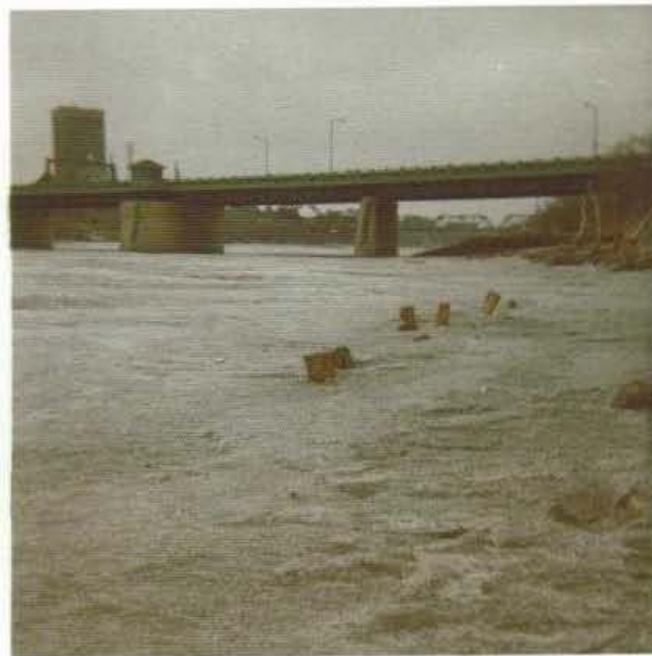
P3.2 Timber pile retard in P3.1 displaced by bank movement, Tache Avenue, 1971.
