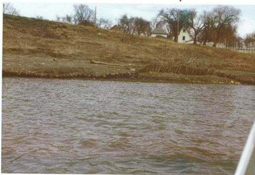
P18. Timber pile retard, closely spaced piles. Note overturning of piles due to bank failure. Red River, 1972.
