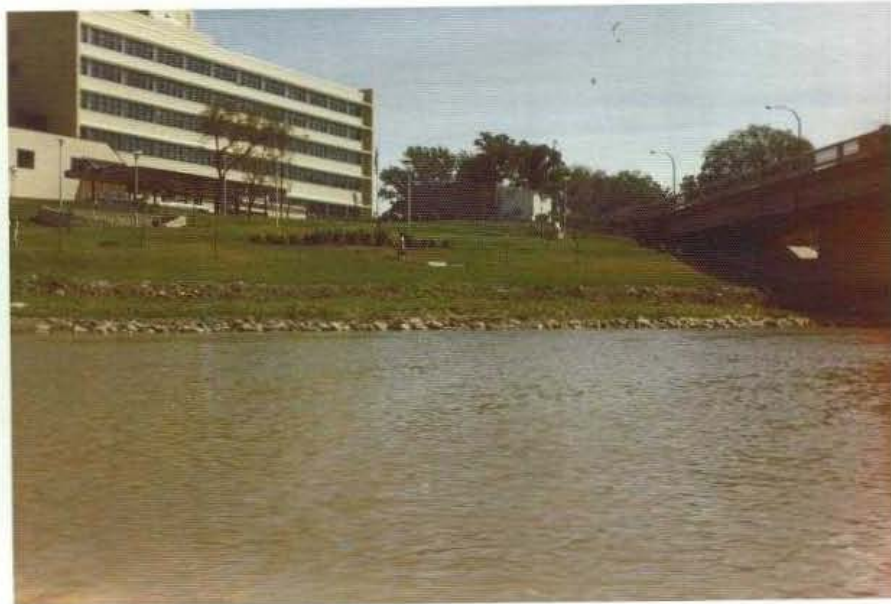
P7. Slope flattening to improve stability with riprap at the toe for erosion protection, Assiniboine River, 1972.
