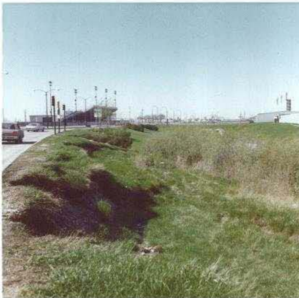
P22.1 Bank failure in backfilled portion of an old channel. Cmands Creek, 1970.
