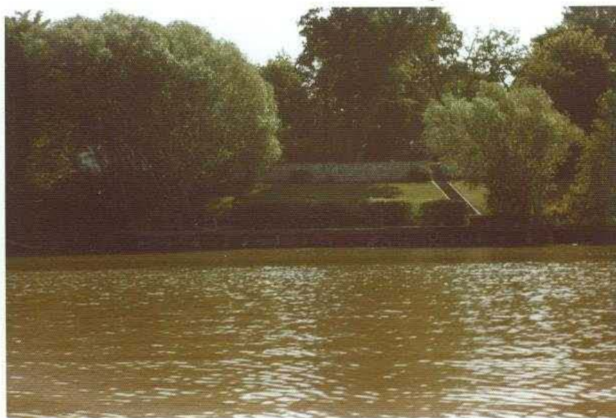
P20. Timber pile retard with horizontal planking. Note stone retaining wall well up the slope. Red River, 1972.
