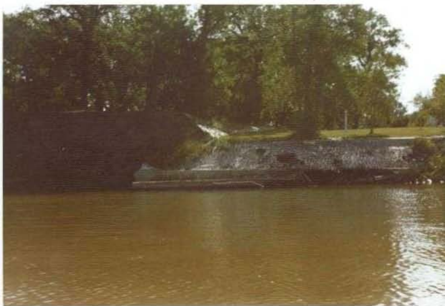
P12 Rigid revetment for slope protection. Note failure of revetment on the right. Red River, 1972.
