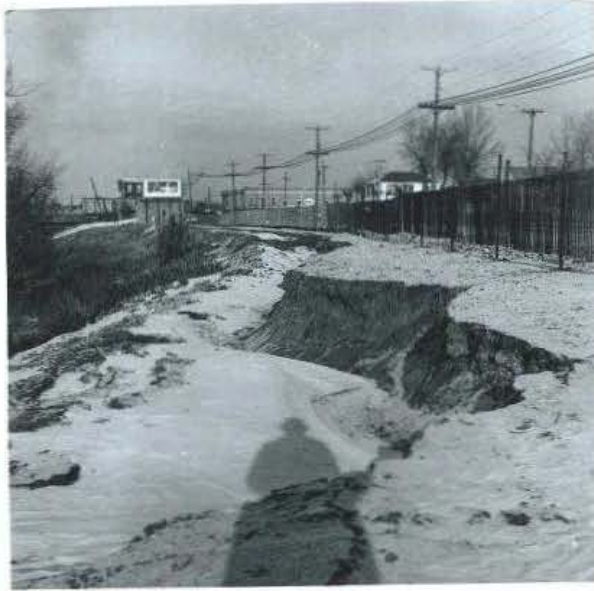
P4.1 New failure scarp, Tache Avenue site, 1959.
