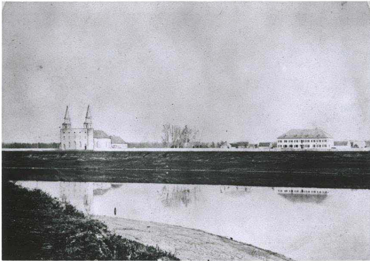
P2. Tache Avenue riverbank site, 1858. Note what appears to be a fresh failure scarp. Courtesy Manitoba Provincial Archives.
