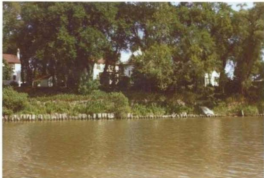
P16. Timber pile retard, piles closely spaced. Red River, 1972.
