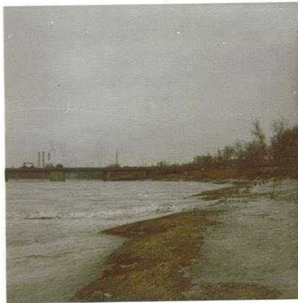
P6. Example of an overthrust of soil at the toe of the failure, Tache Avenue, 1971.
