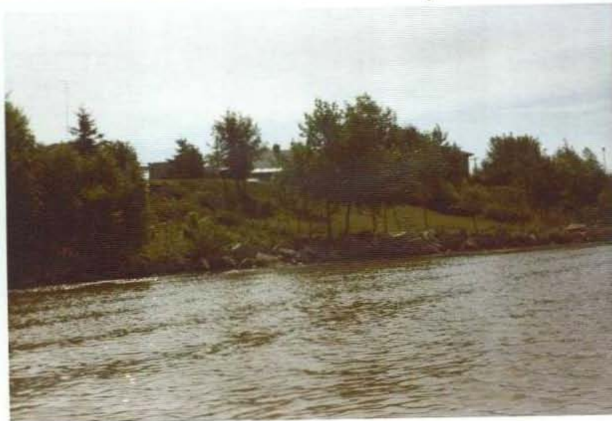
P11. Riprap protection to just above summer water level. Note size and gradation of riprap. Red River, 1972.
