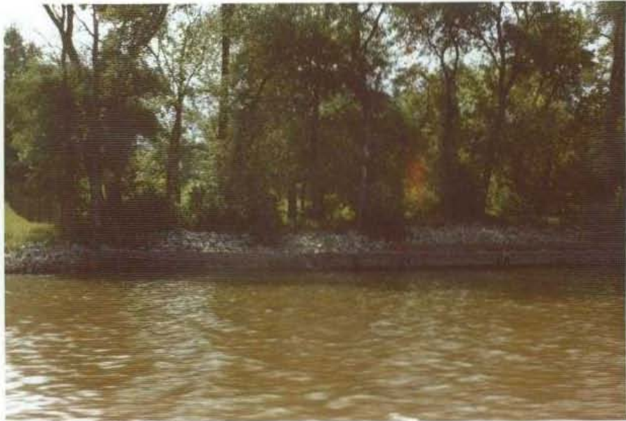
P13. Combination of timber piling retard and riprap slope protection, Red River, 1972.
