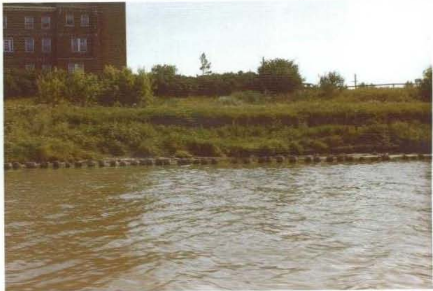
P15. Timber pile retard, single pile spacing. Note condition of bank behind retard. Red River, 1972.
