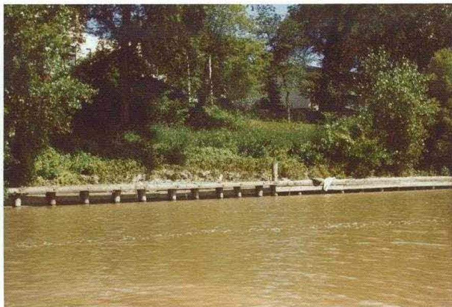
P19. Timber pile retard with horizontal planking. Assiniboine River, 1972.
