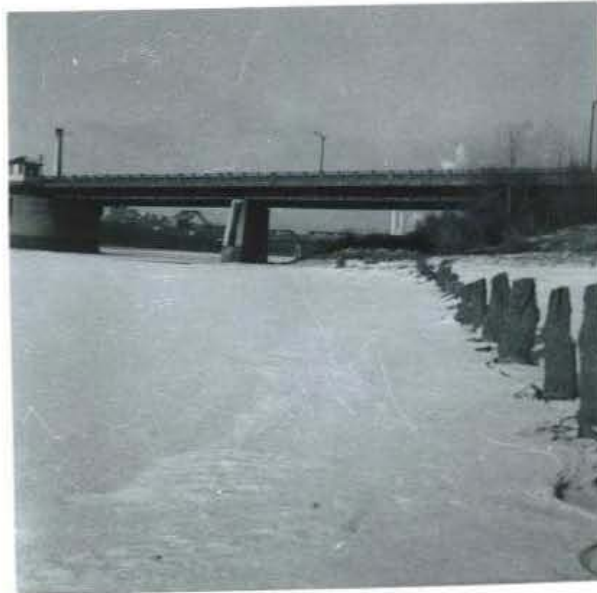
P3.1 Timber pile retard at toe of slope. Tache Avenue riverbank, 1959.
