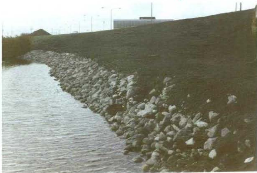
P10. Riprap protection to just above summer water level, Omands Creek, 1972.
