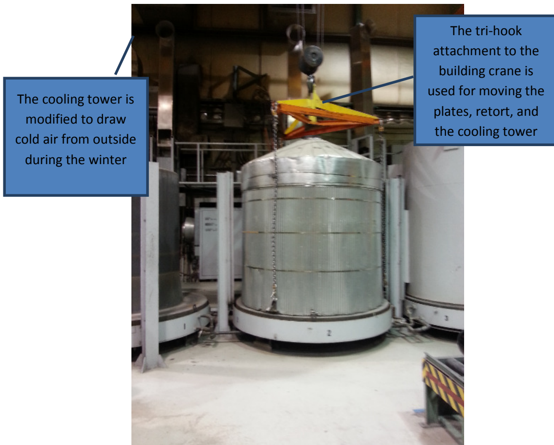
Figure 7: Cooling tower external view
