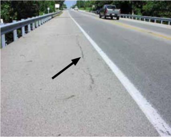
(a) Asphalt overlay longitudinal cracking
