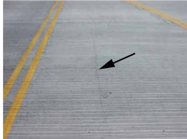
(b) Concrete topping longitudinal cracking
