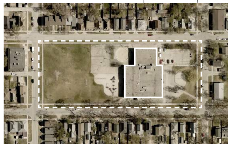
Fig. 48: Existing school condition (Lins, 2020)
