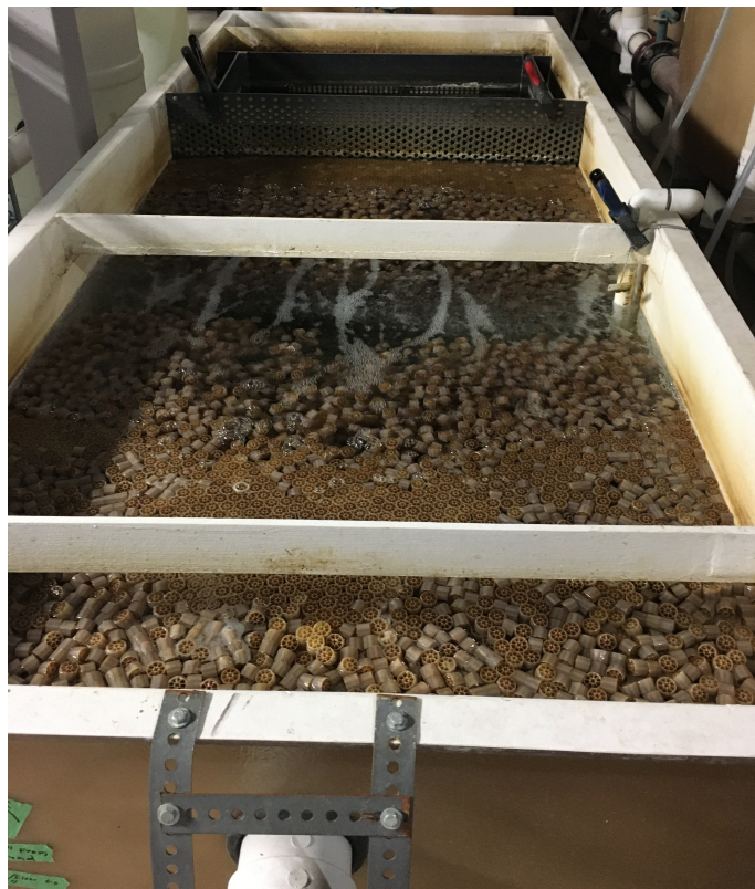
Figure 4.4: RAS biofilter is filled with growth media on which nitrifying bacteria reside. They convert ammonia and ammonium in the water into nitrates, which are safer for the fish. The bubbles in the middle of the tank are from a submerged air-pump which ensures there is enough oxygen supply available to the bacteria.
