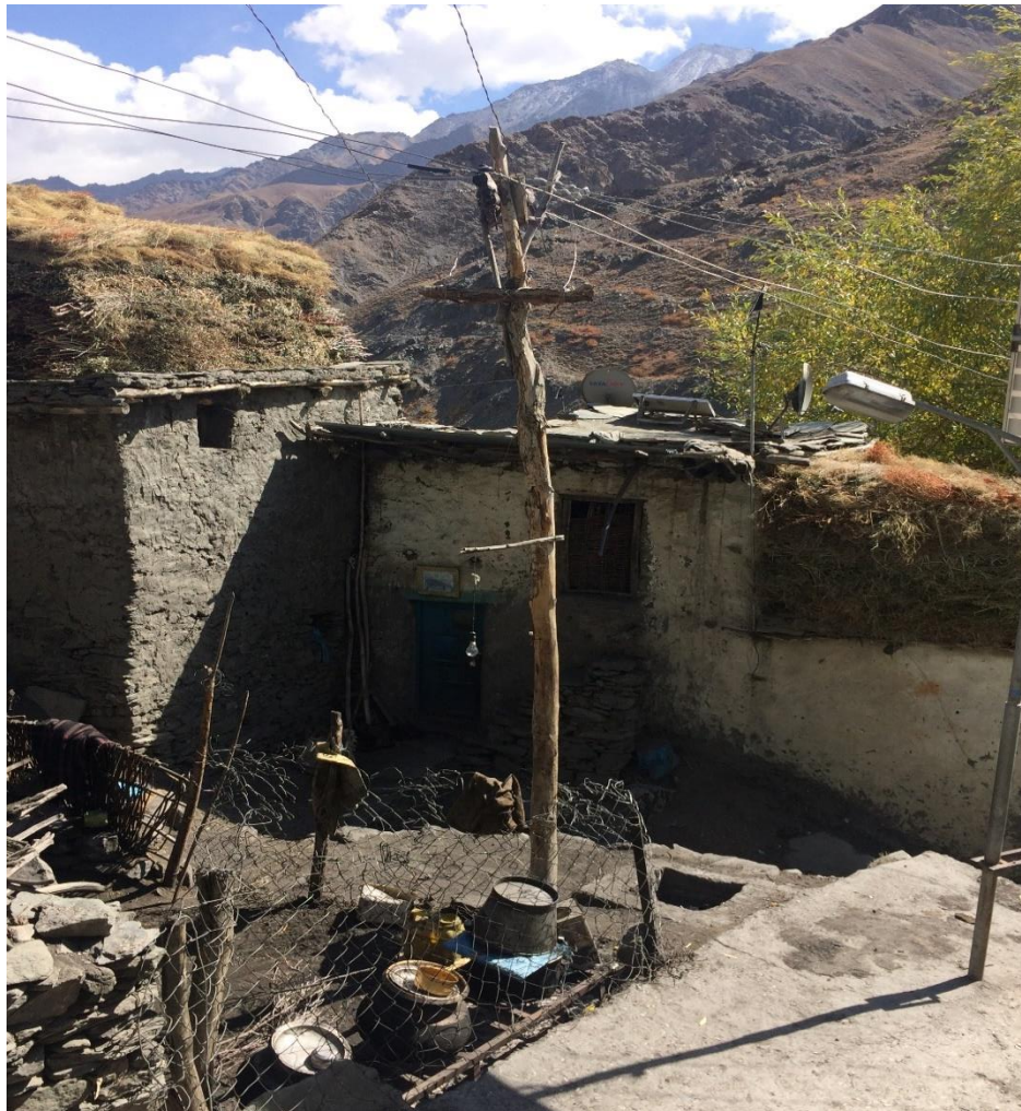
Figure 29: Locally Fabricated Wooden Pole, Bartoo (Source: Gurmeet Singh Ghera)
