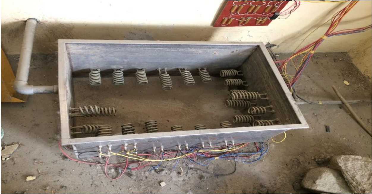
Figure 12: Water Heating System at the Project (Source: Gurmeet Singh Ghera)
