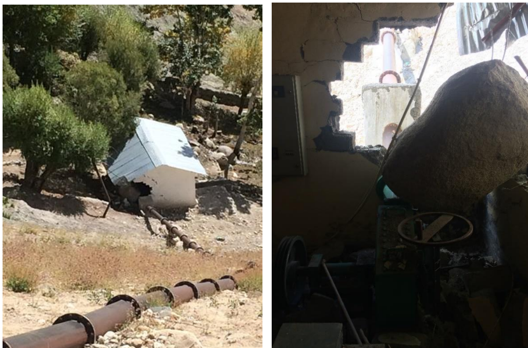
Figure 26: Damage to the Power House due to Rock Fall, Yangthang (Source: Gurmeet Singh Ghera)
