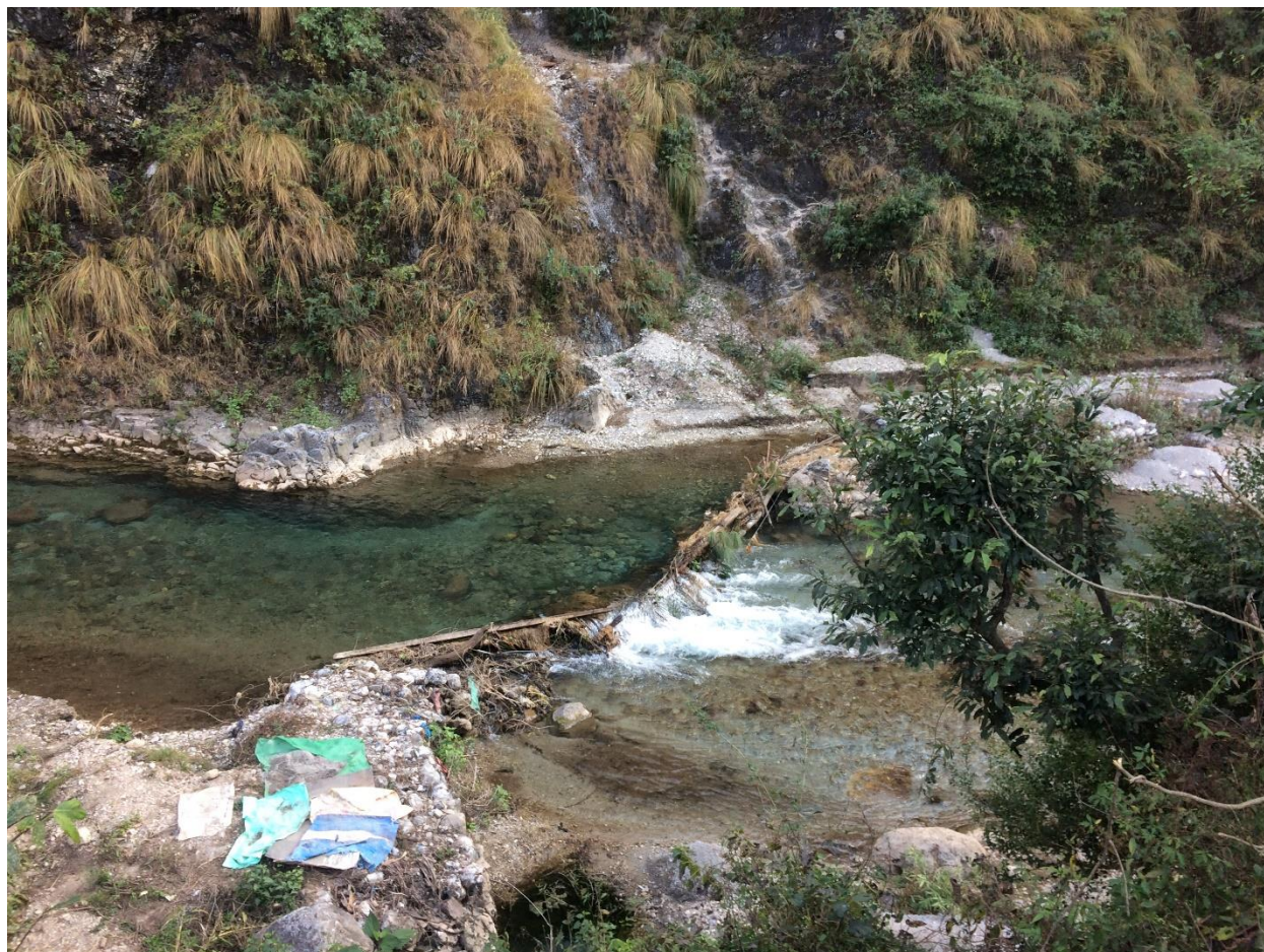
Figure 17: Broken Canal Diversion, Lamabagar (Source: Gurmeet Singh Ghera)
