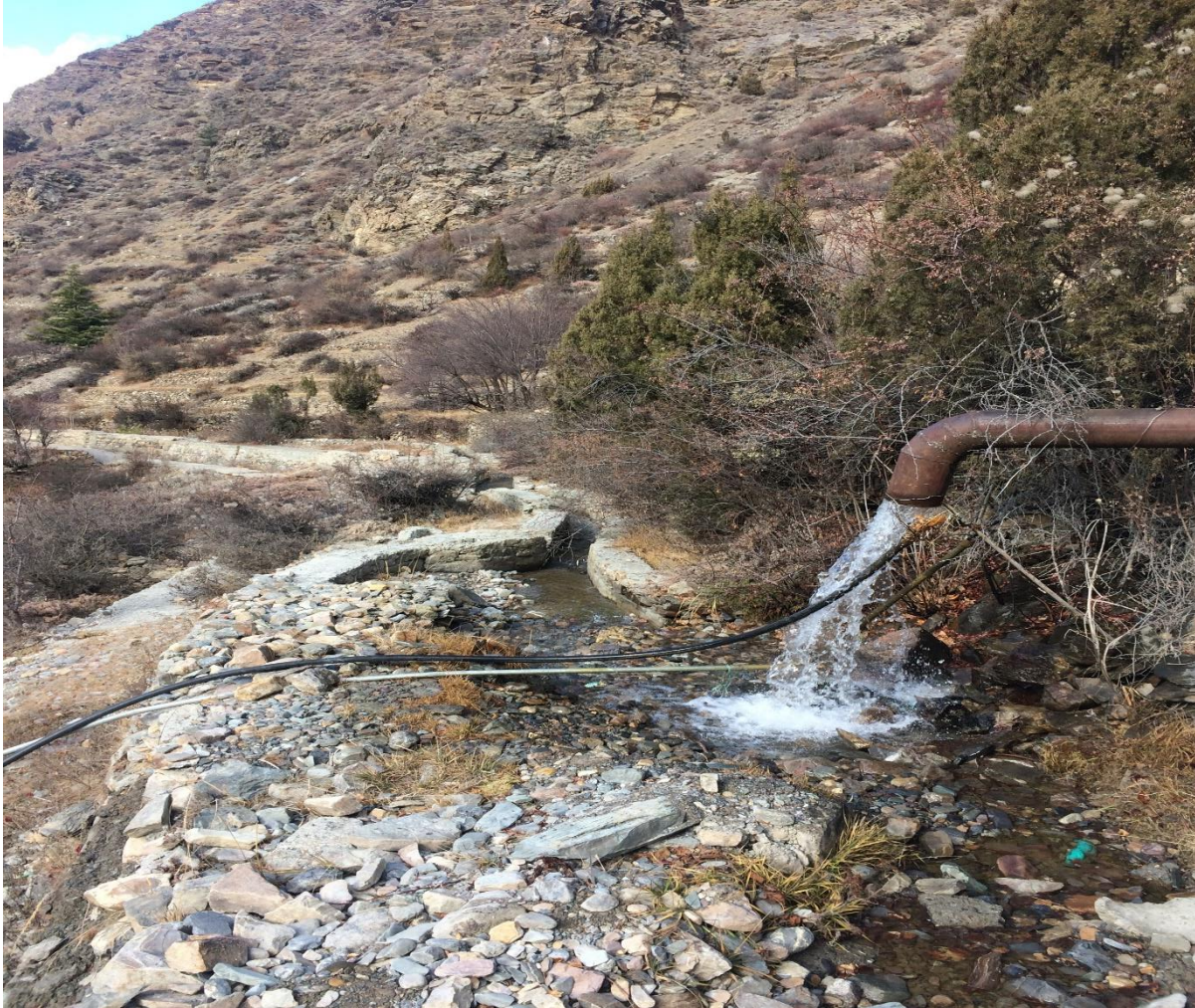
Figure 18: Tailrace feeding the irrigation canal, Malari (Source: Gurmeet Singh Ghera)
