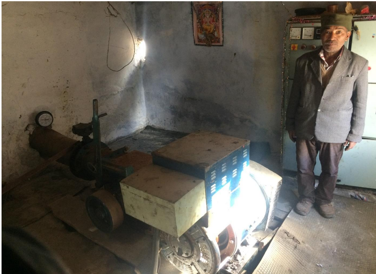
Figure 19: Village Head at the Powerhouse, Malari (Source: Gurmeet Singh Ghera)
