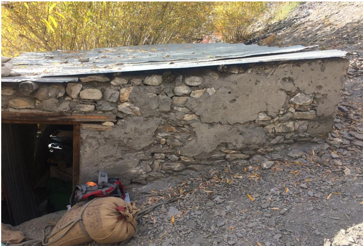
Figure 10: Yarkashing Power House (Source: Gurmeet Singh Ghera)
