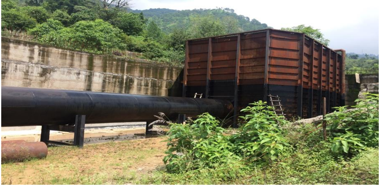
Figure 1: Settling Tank (Source: Gurmeet Singh Ghera)
