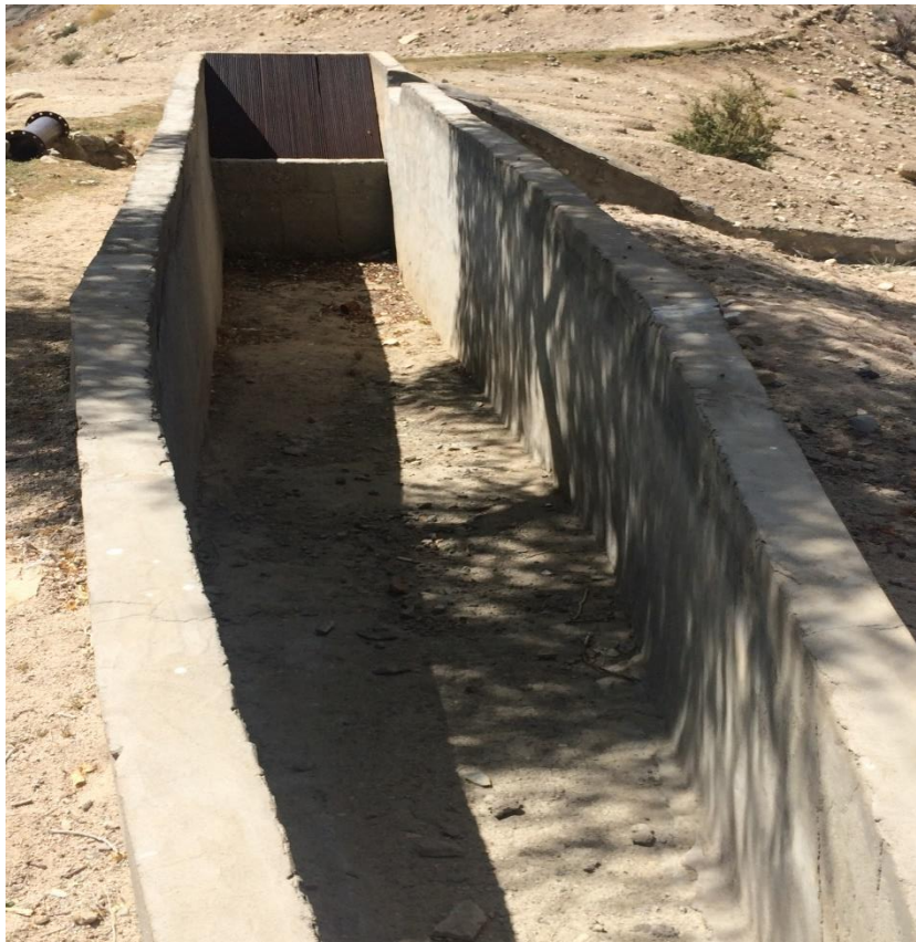
Figure 13: Dry Forebay (Source: Gurmeet Singh Ghera)
