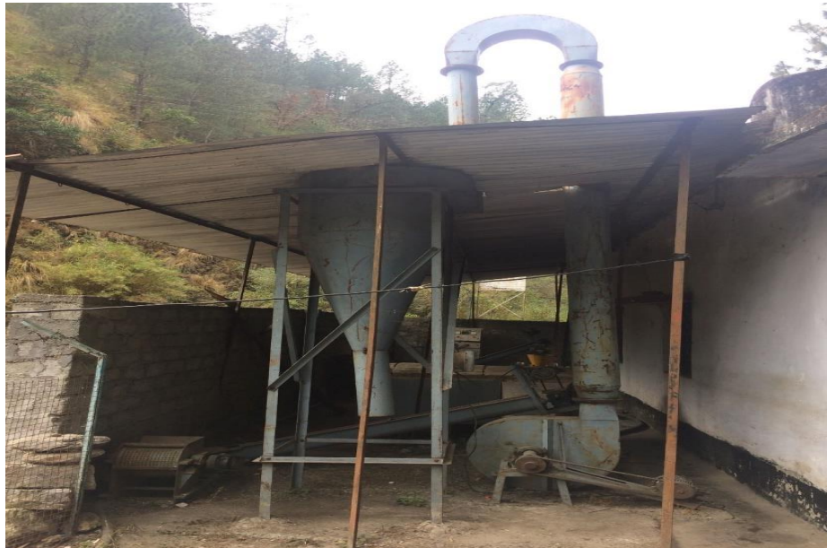
Figure 25: Coal Making Plant, Toli (Source: Gurmeet Singh Ghera)
