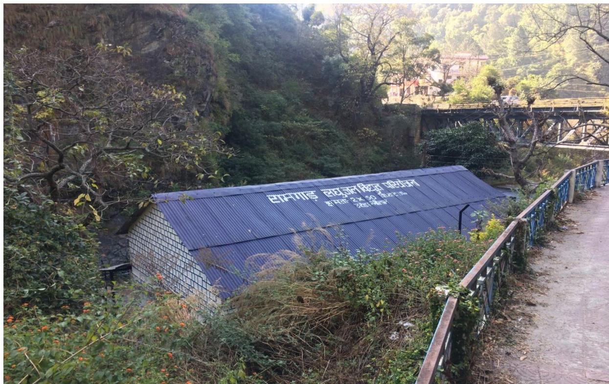
Figure 15: Powerhouse Building, Ramgaad (Source: Gurmeet Singh Ghera)
