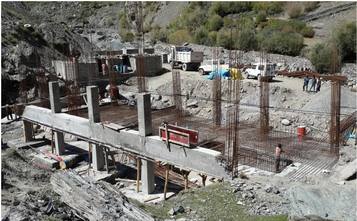
Figure 7: 1.5 MW Khandi Small-Hydro Power Plant Under Construction (Source: LREI Report)
