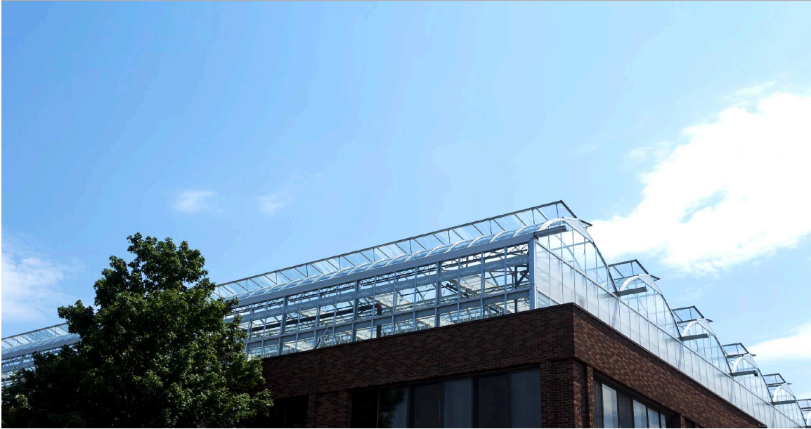
Figure 12: Commercial Case Study - Lufa Farms Ahuntsic Location Rooftop Garden (Lufa Farms, 2018, p. 9).
