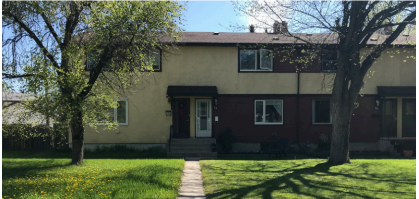
FIG 4.63 Top. This building shows a beige facade that features three different materials. The front yard has a number of trees and planting beds.
