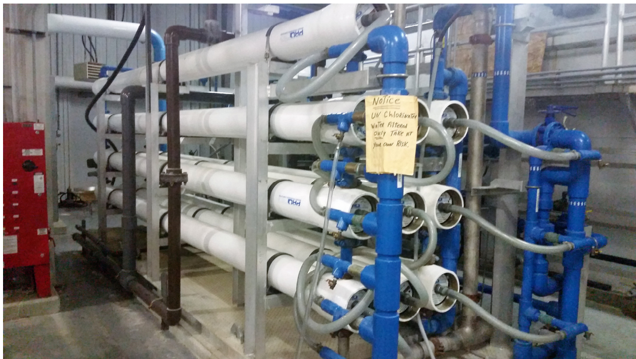
Figure 58: Photo of RO membrane system at the Pine Creek First Nation WTP showing a note stating, "unchlorinated water filtered only take at own risk." Picture was taken in January 22, 2015.
