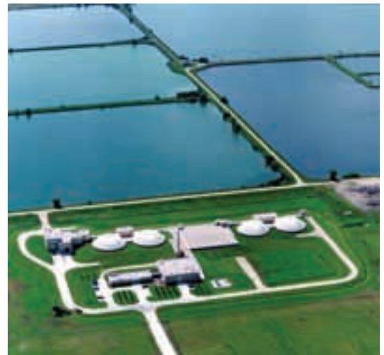
The City of Winnipeg's west end wastewater treatment plant.
