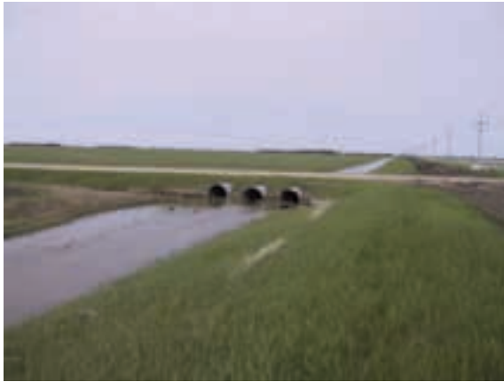
Agricultural drainage networks are designed to move snowmelt and rainfall runoff water from fields.
