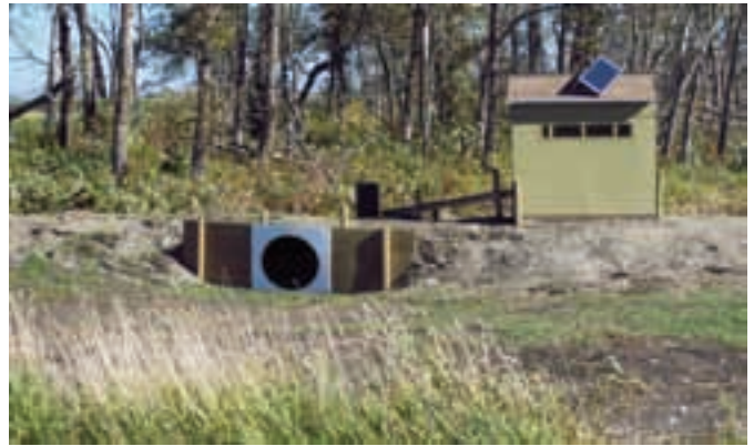
Watershed Evaluation of Beneficial Management Practices project in the South Tobacco Creek watershed.
