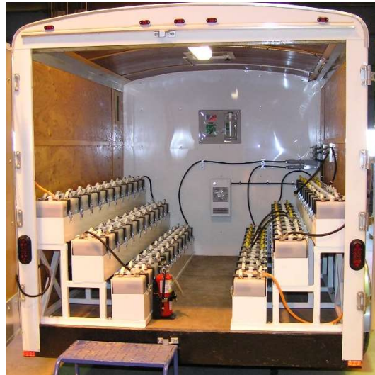
Figure 2.5 Station (133 V) and communication (48 V) mobile trailer. 3
