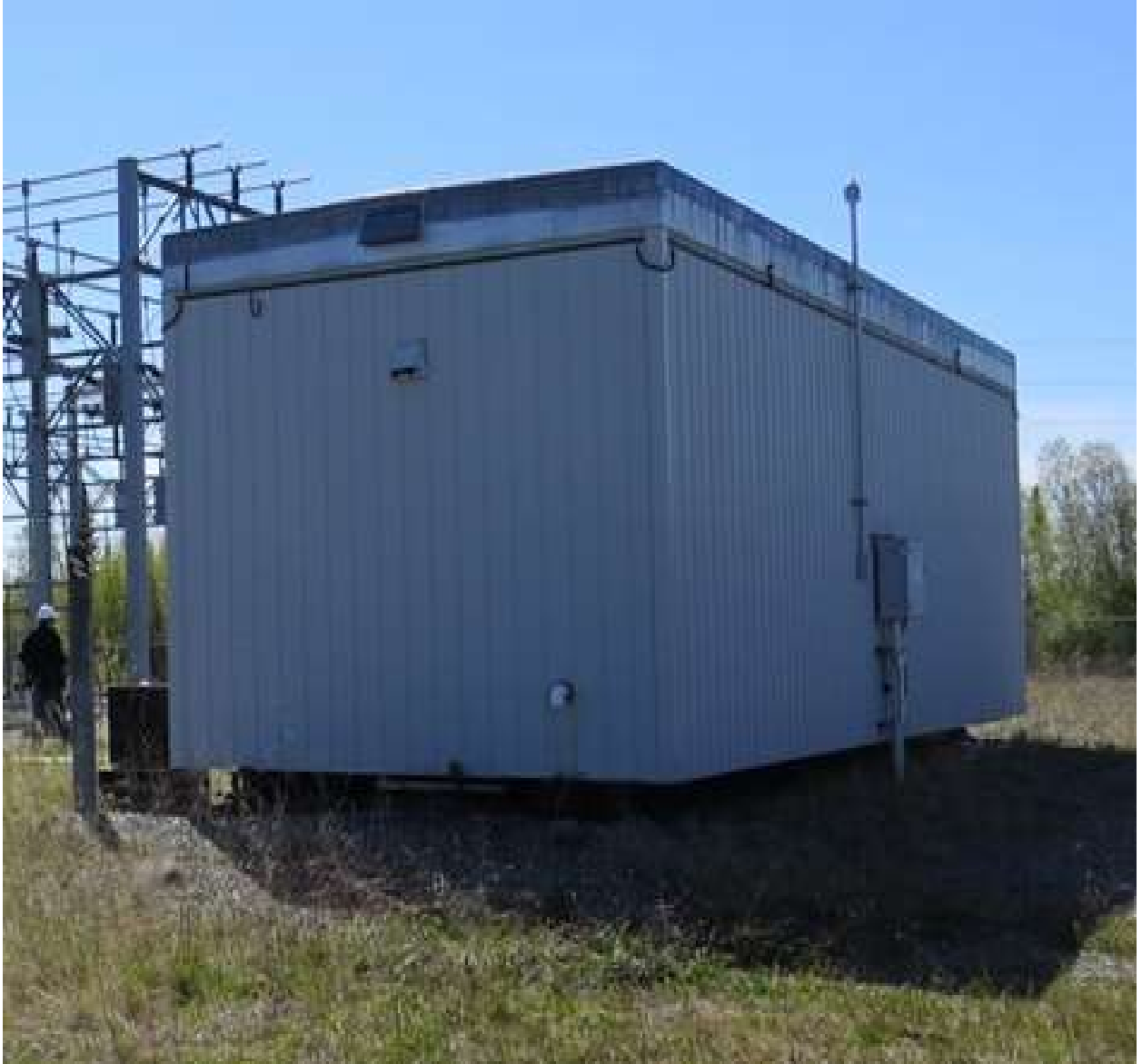
Figure 1.1.1 Ready to move trailer 1
