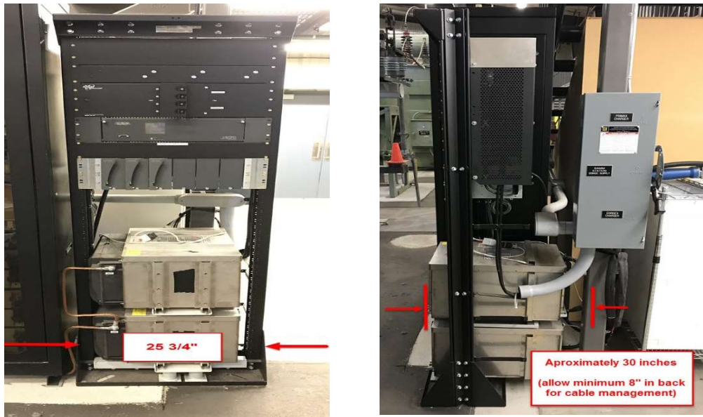
Figure 4.3 Stonewell sodium-nickel-chloride experimental setup
