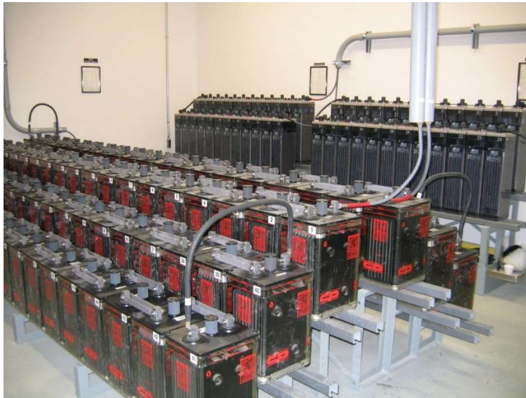
Figure 2.17 Substation battery bank 4
