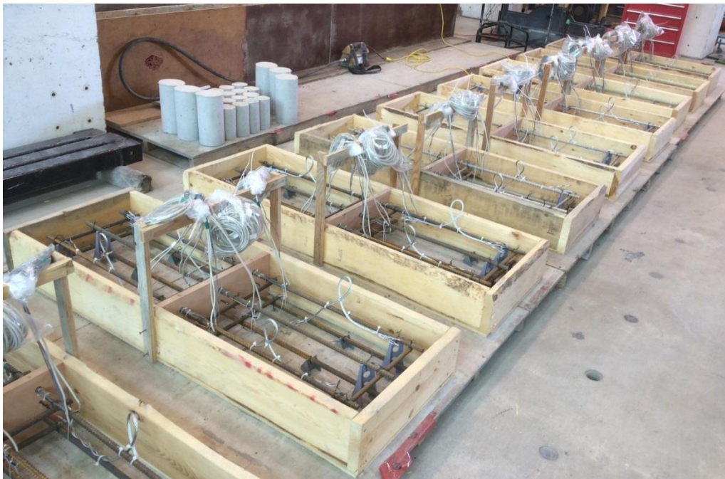
Figure 32 Formwork prior to casting
