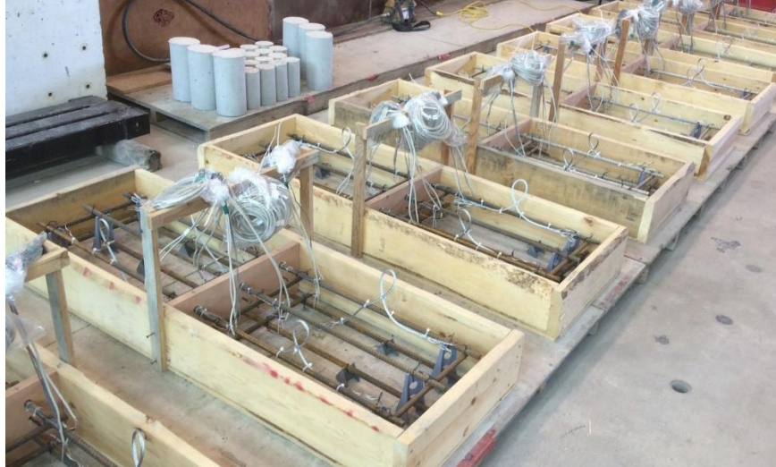
Figure 20 Formwork prior to casting including thermal sensors
