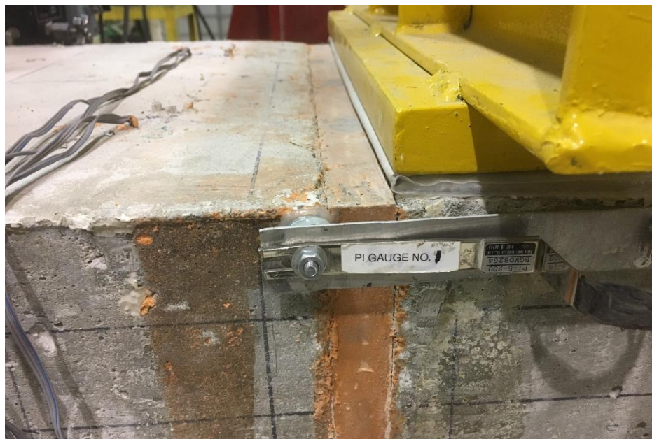
Figure 67 Image of sample number 10 showing minimal opening of the thermal break prior to steel yielding
