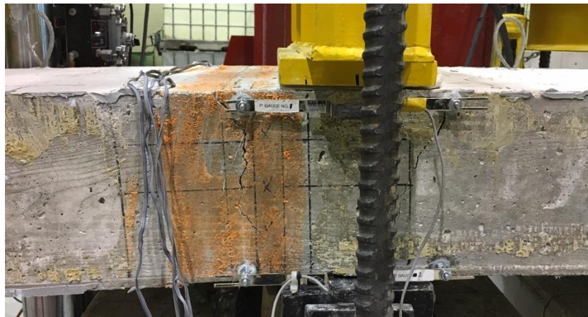
Figure 70 Sample number 8 after yielding of the steel reinforcement
