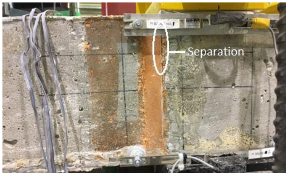
Figure 72 Sample 13 prior to yielding of the stainless steel reinforcement
