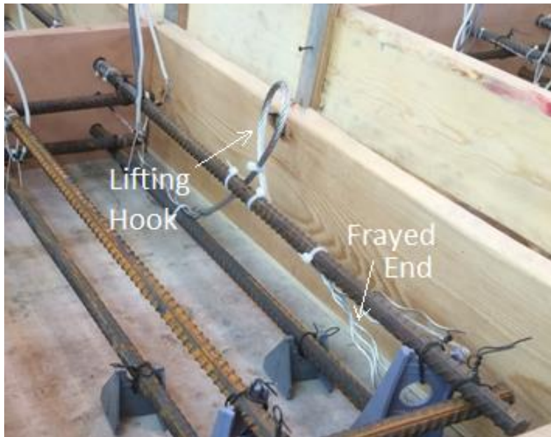
Figure 34 Lifting hook attached to reinforcing bar in formwork
