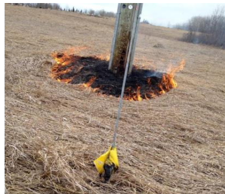
Photo 2 and 3: Fire damaged hydro pole and prescribed burn around hydro pole in WIN. Source: (OMNRF)
