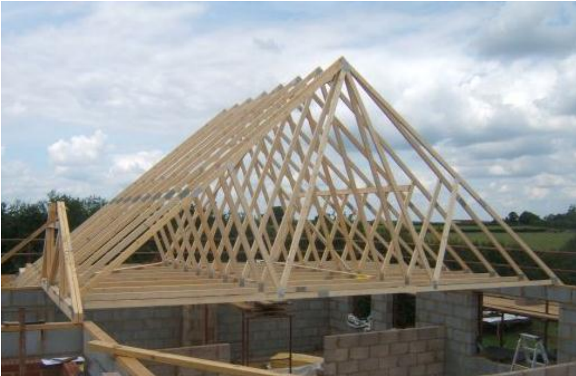
Figure 2: Truss Placement Elaboration Source: Vision Development
