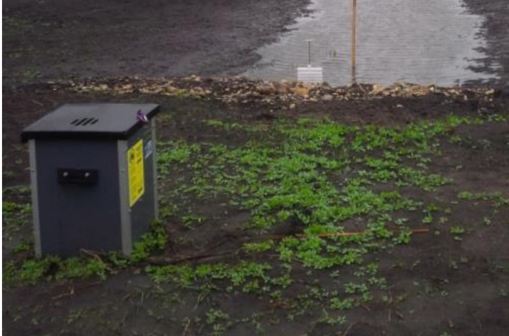
Figure 2.16. Agridrain control structure at retention pond outlet and inlet into site B3, May 2015
