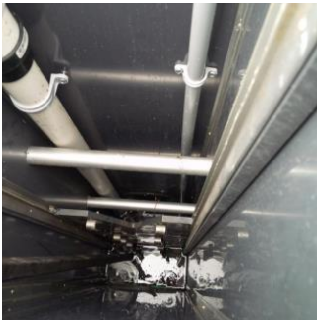
Figure 2.17. Inside of Agridrain control structure at retention pond, inlet into site B3, May 2015
