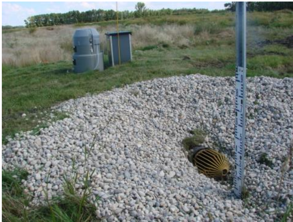
Figure 2.15. Outlet pipe through berm at site B1, August 2016
