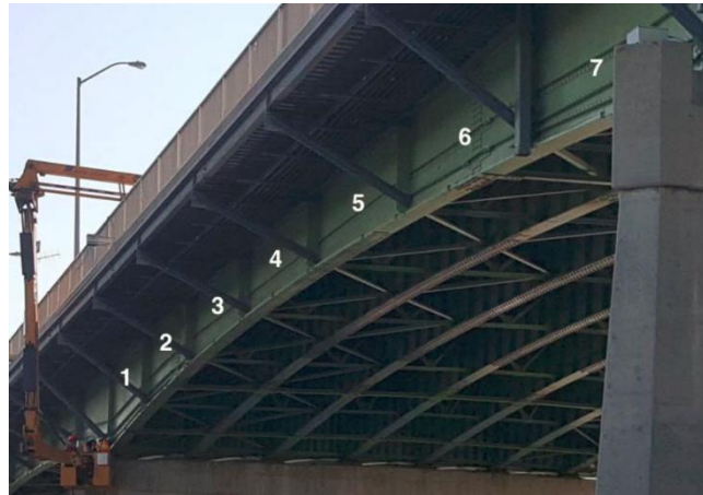
Figure 5. 10. Installation of binary crack sensor on a 30-meter span steel girder of a bridge in 7 segments.
