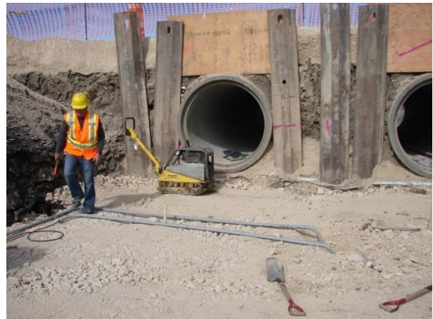
b) L-shaped Thermistor String.
