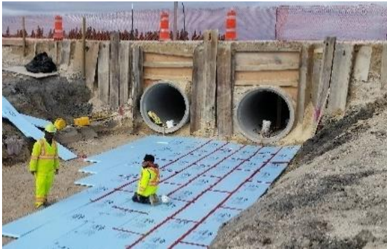
Figure 3.5: Rigid insulation placement under the culverts at site 3
