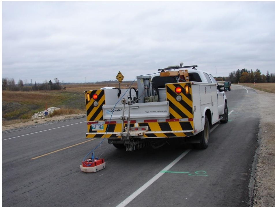
Figure 3.10: Performing 400MHz GPR scan over Site 4
