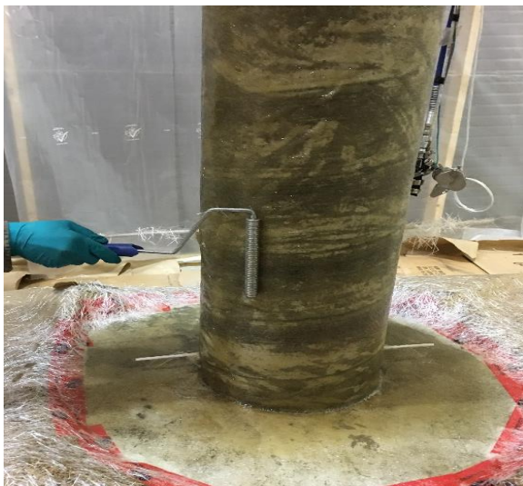
(c) Entrapped air removal
