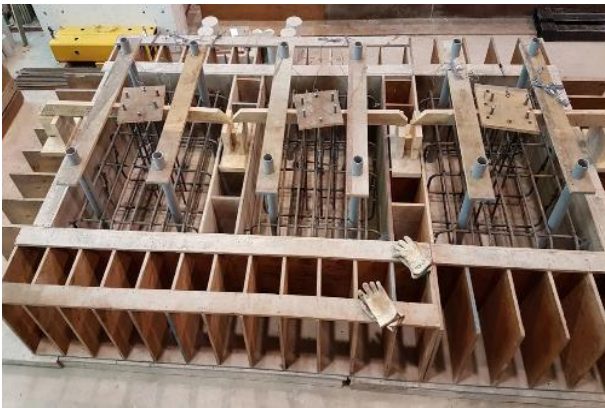
(a) Steel cages for column footings
