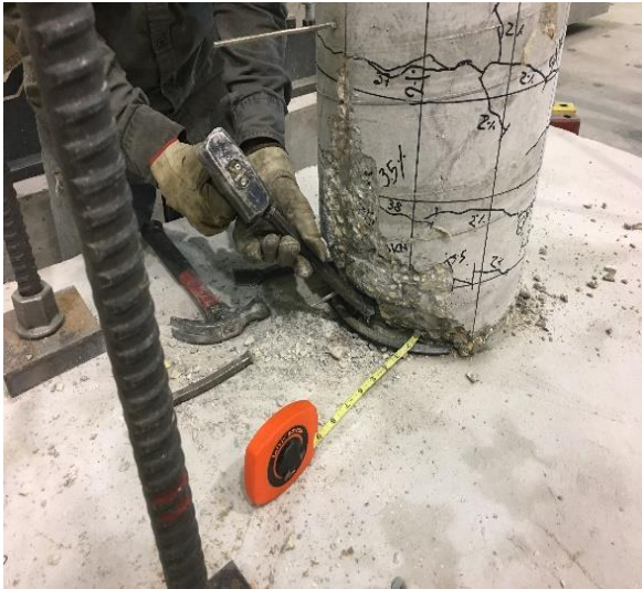
(a) Removing loose and spalled concrete
