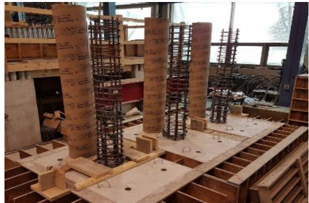
(b) Casting footing with column reinforcement
