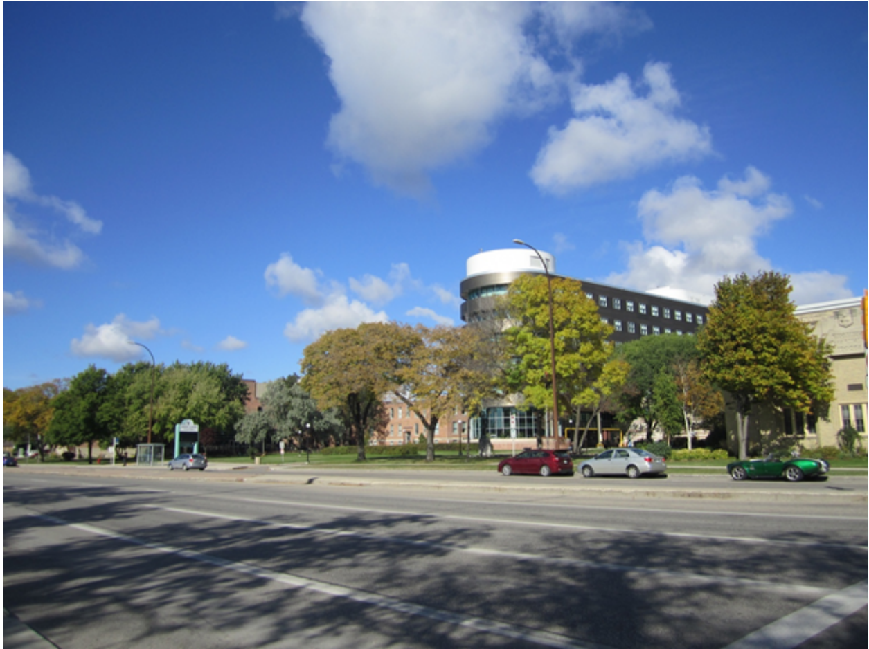
Figure 10: Deer Lodge Centre: A view of the campus, highlighting the central building that functions as a focal point and way-finding beacon for the site.
