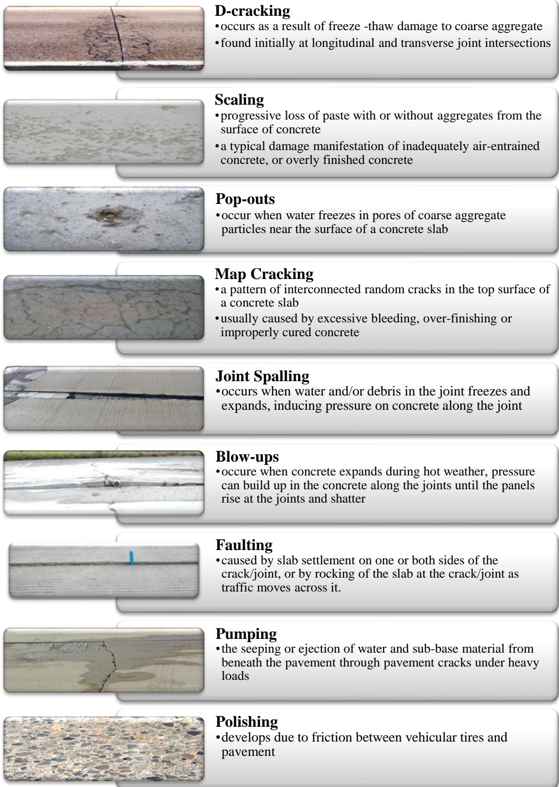
Figure 2.2: Various damage manifestations in concrete pavements (definitions are extracted from Harrington et al. 2014; Shahin 2005; Rangaraju 2002; Fang 2001).
