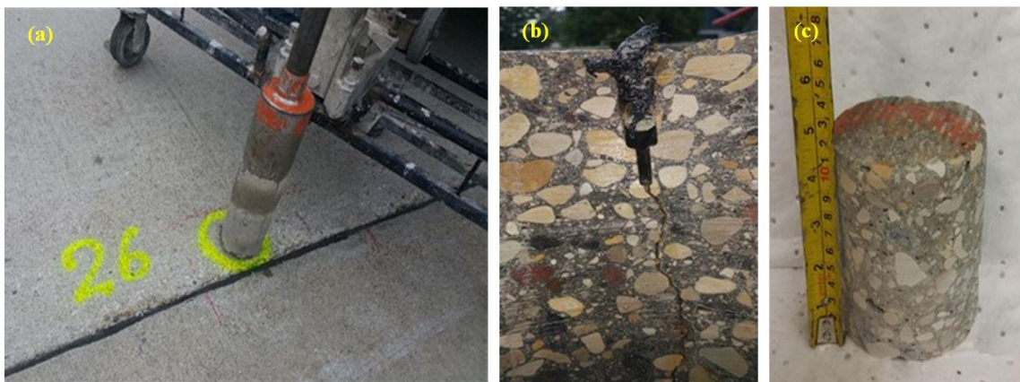
Figure 3.4: An example from a residential street showing: (a) sound joint without evidence of faulting or spalling, (b) joint cross-sections without damage, and (c) whole/intact core.
