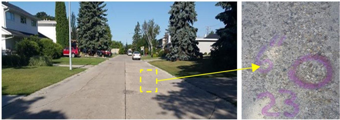
Figure 3.3: A residential street showing surface scaling of concrete.
