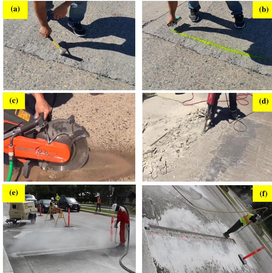
Figure 10.1: Preparation of the transverse joints before repair.
