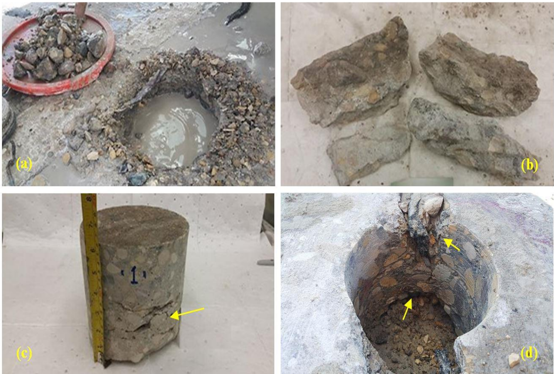
Figure 3.2: An example from regional roads showing: (a) damage of concrete during the coring process, (b) fractured cores, (c) sub-parallel cracks in the extracted cores, and (d) damage of top and bottom parts.
