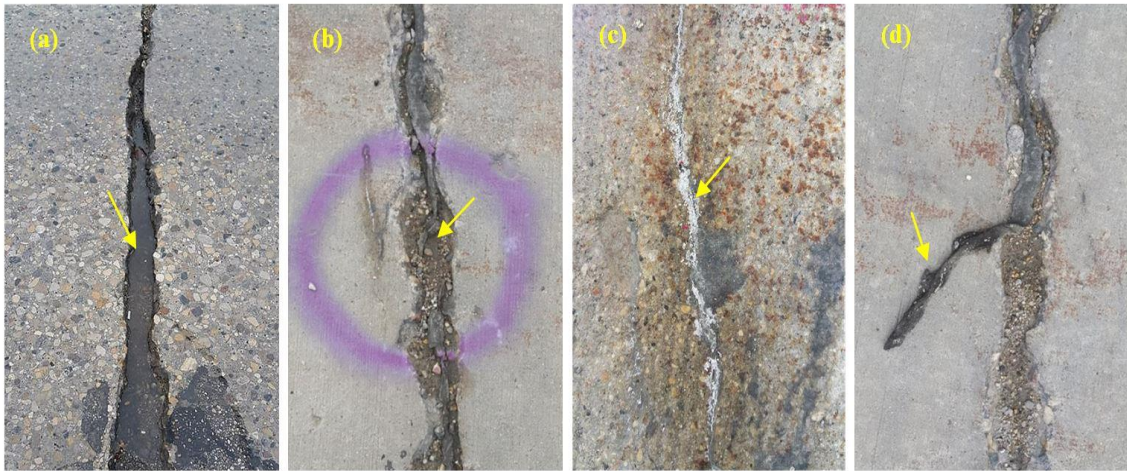
Figure 3.1: Evidence of joint deterioration in regional roads: (a) widening of joints and entrapment of water/solution, (b) shadowing near the joints, (c) cracks filled with white efflorescence, and (d) de-bonded sealants
