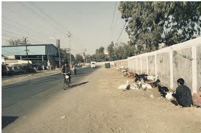
Roadside view of the entrance boundary wall
