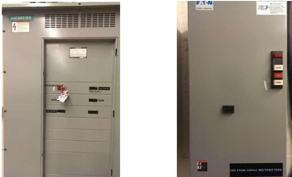
Figure 3.9 Main power supply
