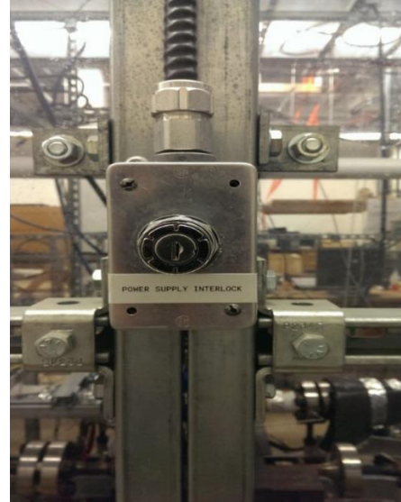
Figure 3.3 Power supply interlock
