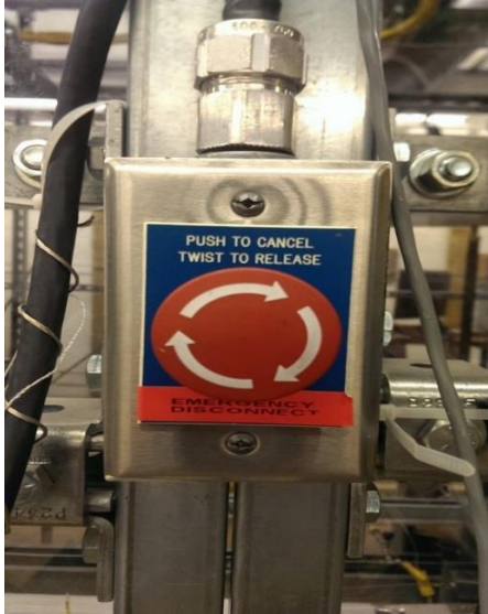
Figure 3.2 Emergency shut down switch
